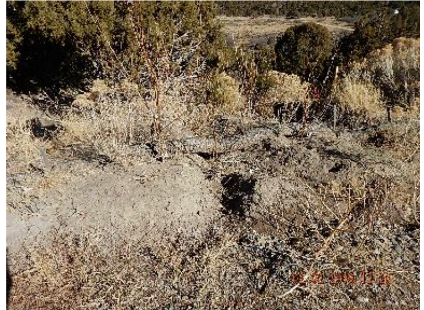
Photo 8: Breach in berm and undercut straw waddle.
