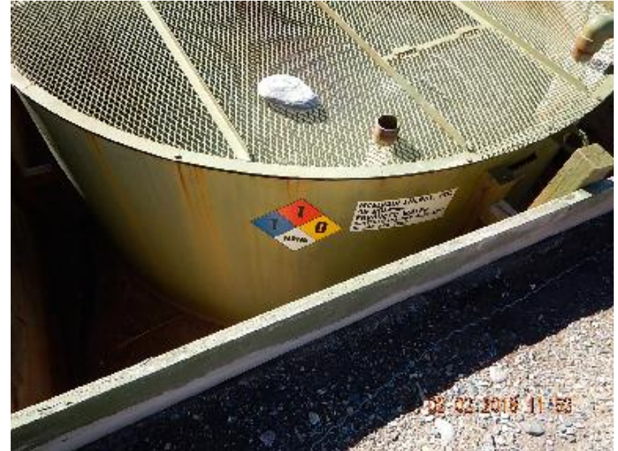
Photo 2: 95 BBL open top tank with below grade labels.
