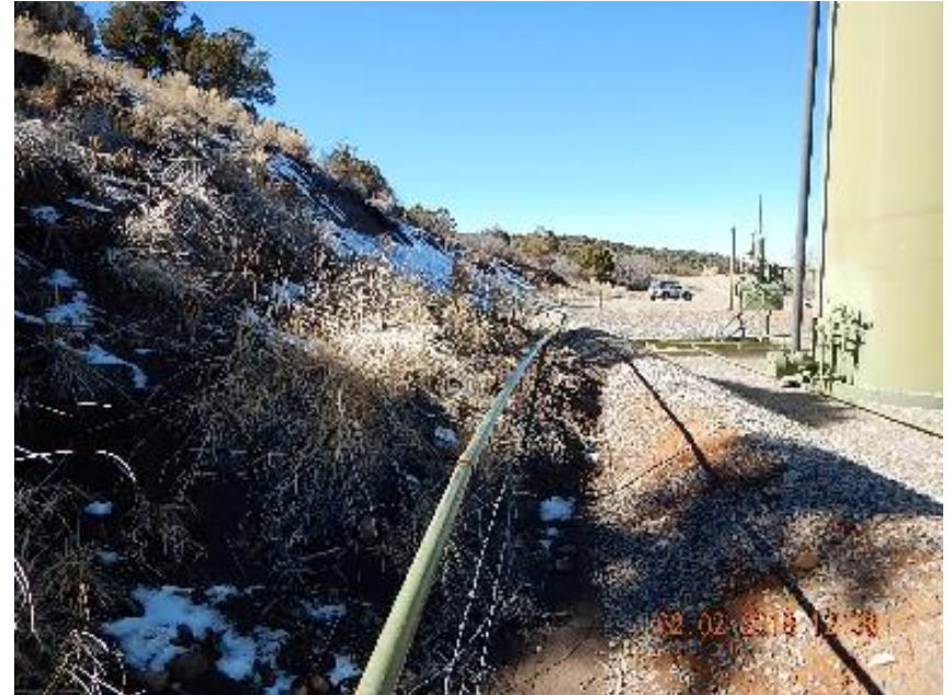
Photo 12: Slide pushing into tank battery fencing.
