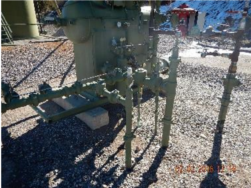
Photo 5: 2" flowline connected at separator.
