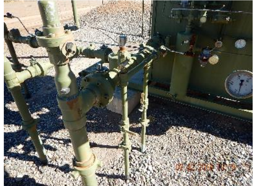
Photo 6: 1" flowline connected at separator.
