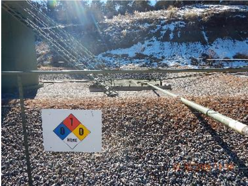
Photo 3: NFPA label on tank battery fencing does not match any labels on tanks.
