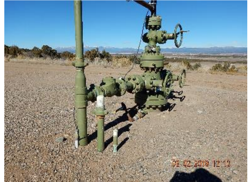
Photo 4: Risers at wellhead for unused 2" and 1" lines.
