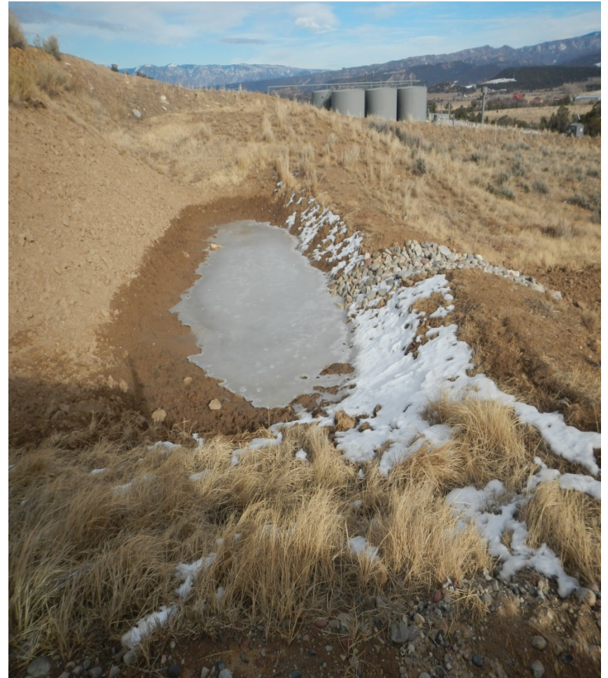
Photo#4: Sediment Trap off East Side of Access Road.
