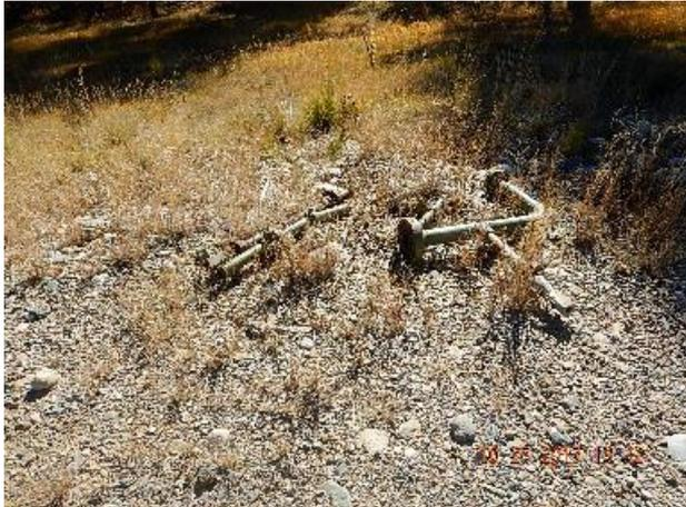
**Photo 13: Disconnected piping on perimeter. Previous inspection.**
