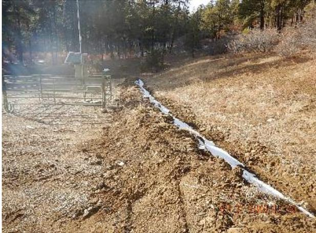
**Photo 17: New ditch and berm at base of cut slope.**
