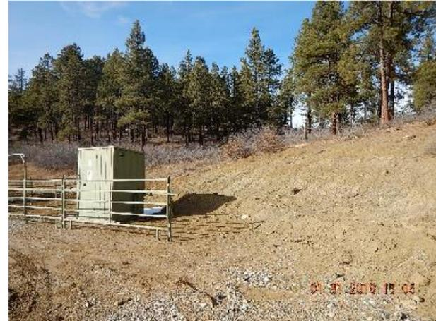
**Photo 8: Repaired cut slope and new ditch and berm.**
