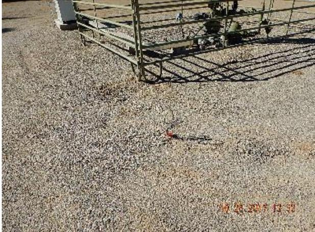
**Photo 15: Wire rope coming out of the ground outside of wellhead fencing. Previous inspection.**
