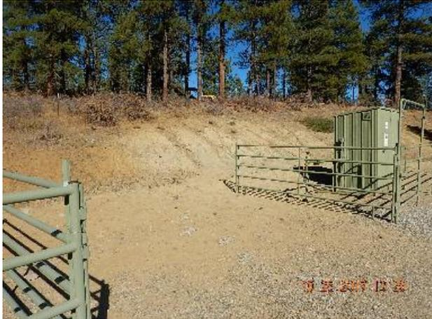
**Photo 5: Erosion rilling with sediment flow onto location in NE corner. Previous inspection.**
