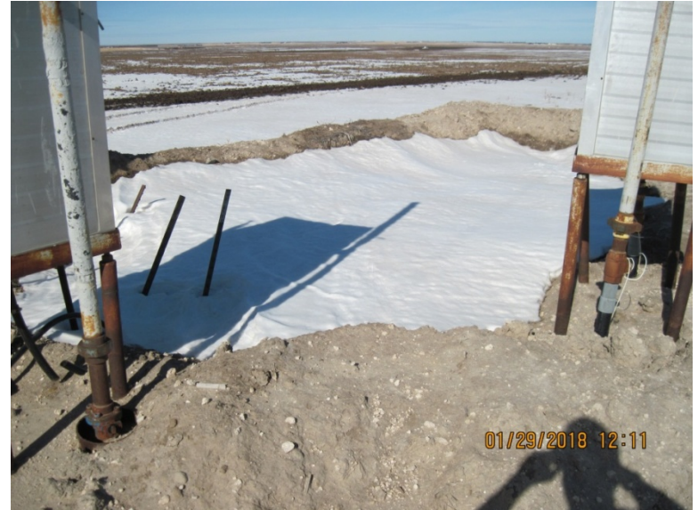
4. Produced water pit
