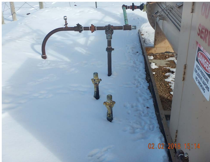
Photo 3: Two marked risers at separator
