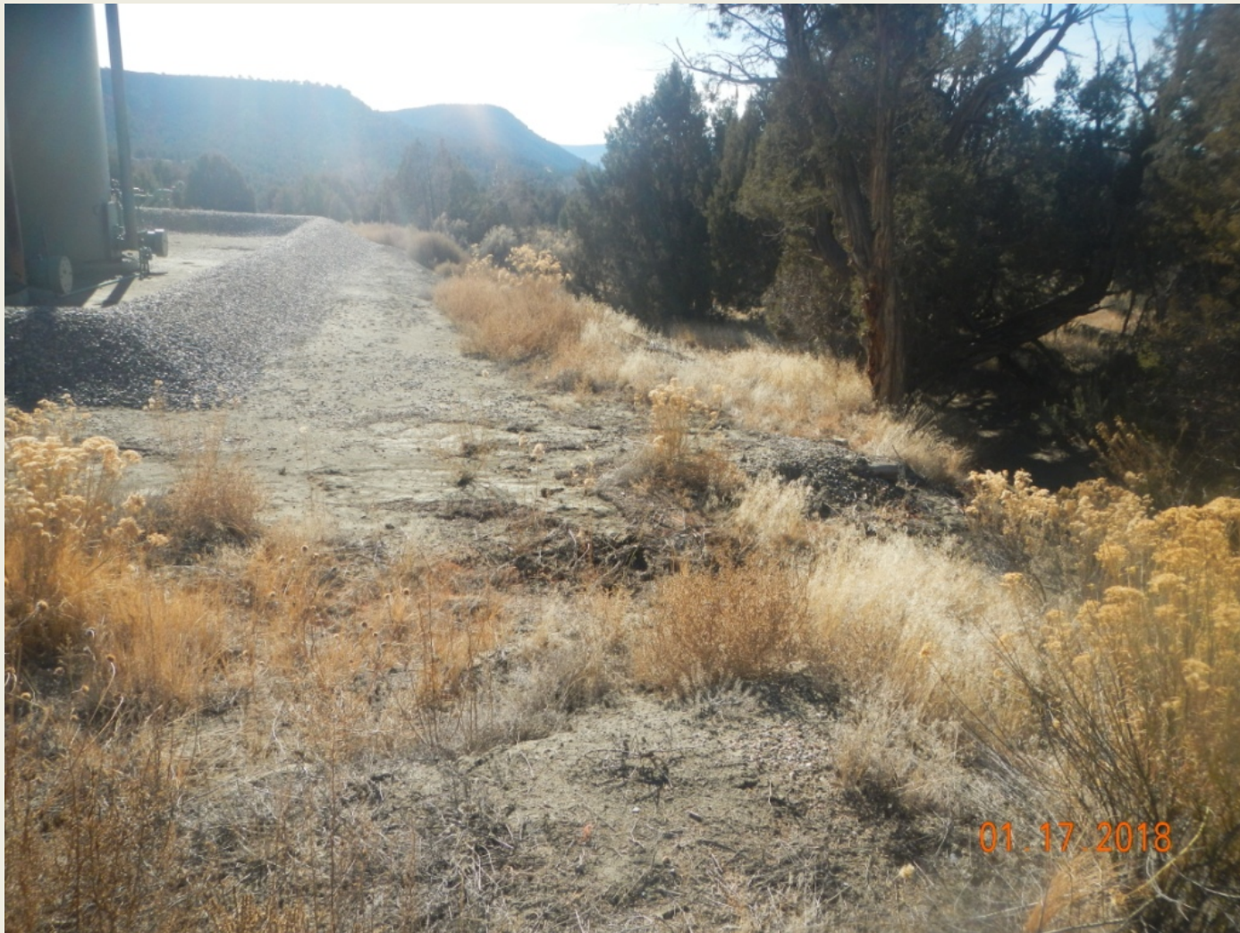
Photo 3. View of the western portion of the project area from northwestern corner facing southward. Erosion is occurring off of the northwestern edge of the well pad.
