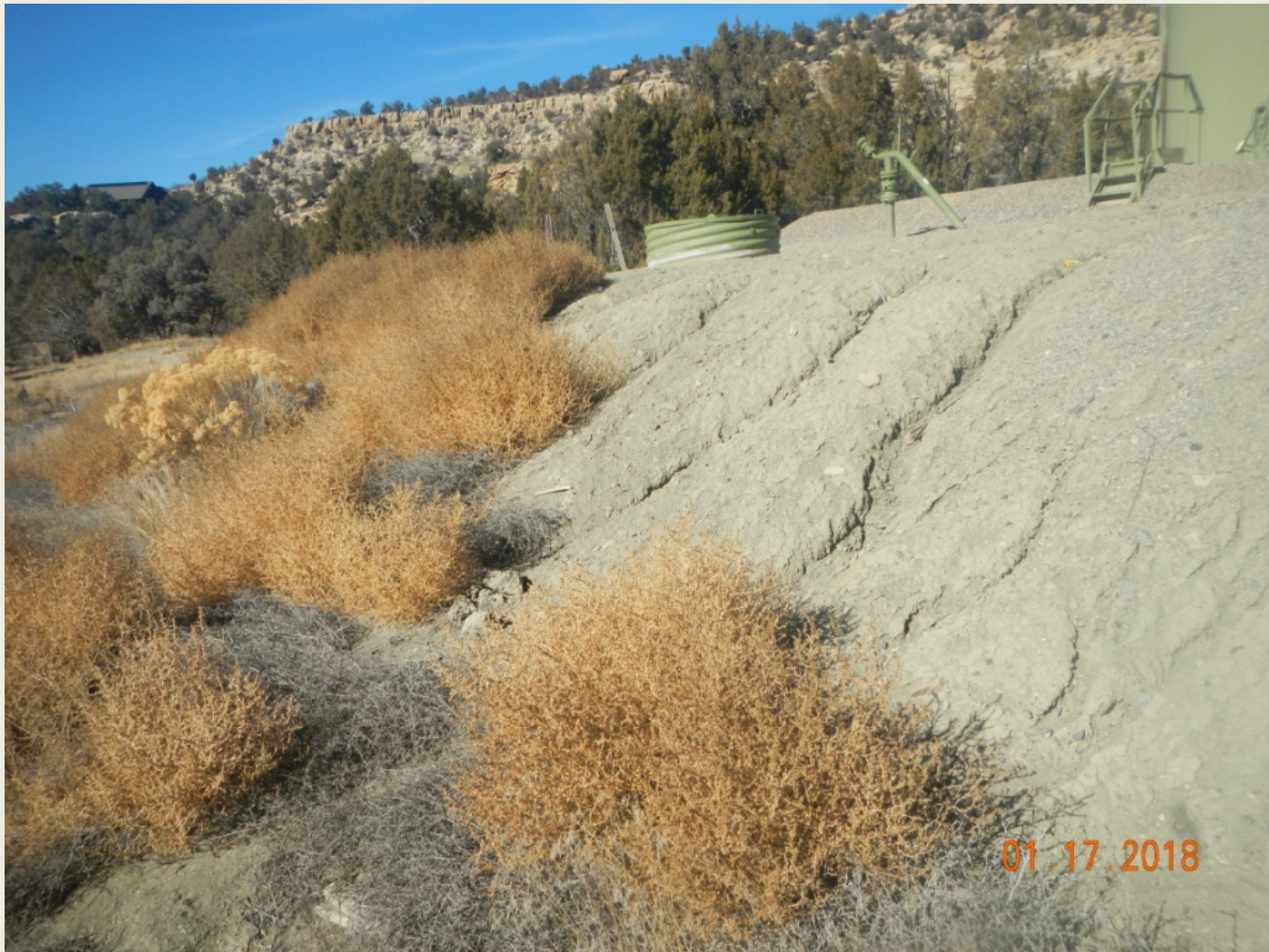
Photo 6. View of erosion channels and Russian thistle ( Salsola tragus ) debris within the southern portion of the project area. This slope needs stabilization, and seeding. R. thistle needs to be removed and properly disposed of.
