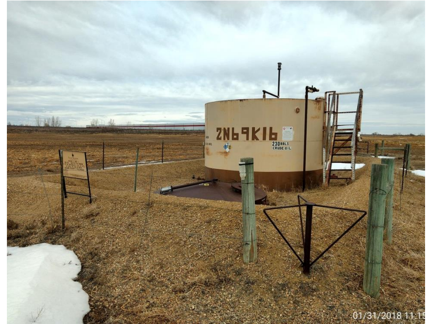
Battery Corrective Action: Unused Enardo valve and piping on top of water tank. Comply with 603.f
