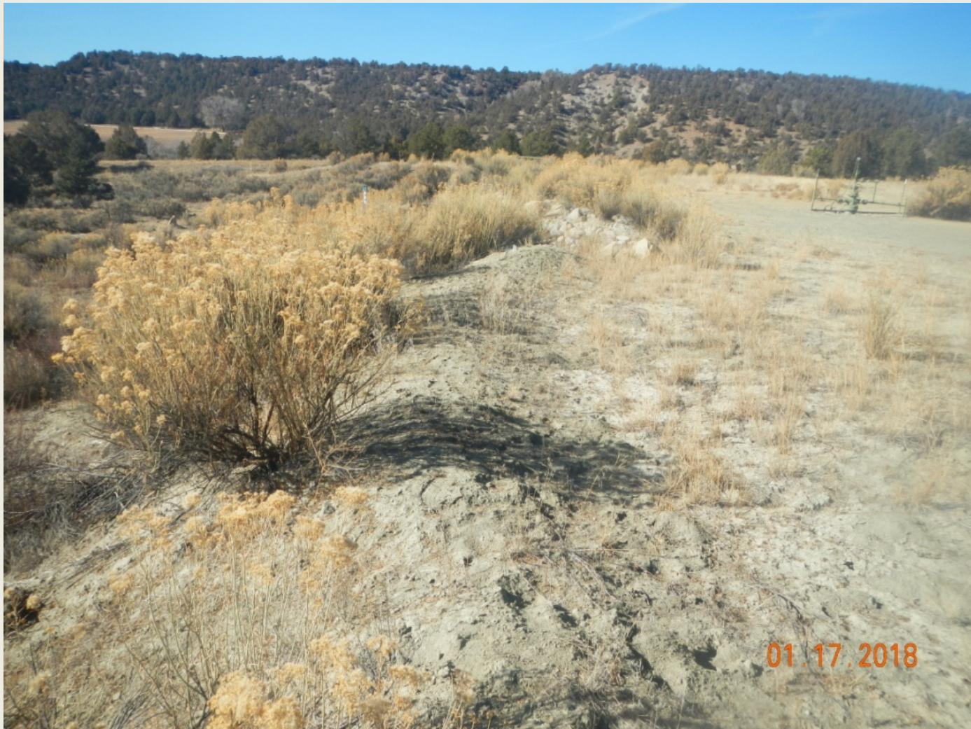
Photo 3. View of the southern portion of the project area from northern corner facing westward. Stormwater controls with cobble run-downs in this portion of the project area appear to be functioning.
