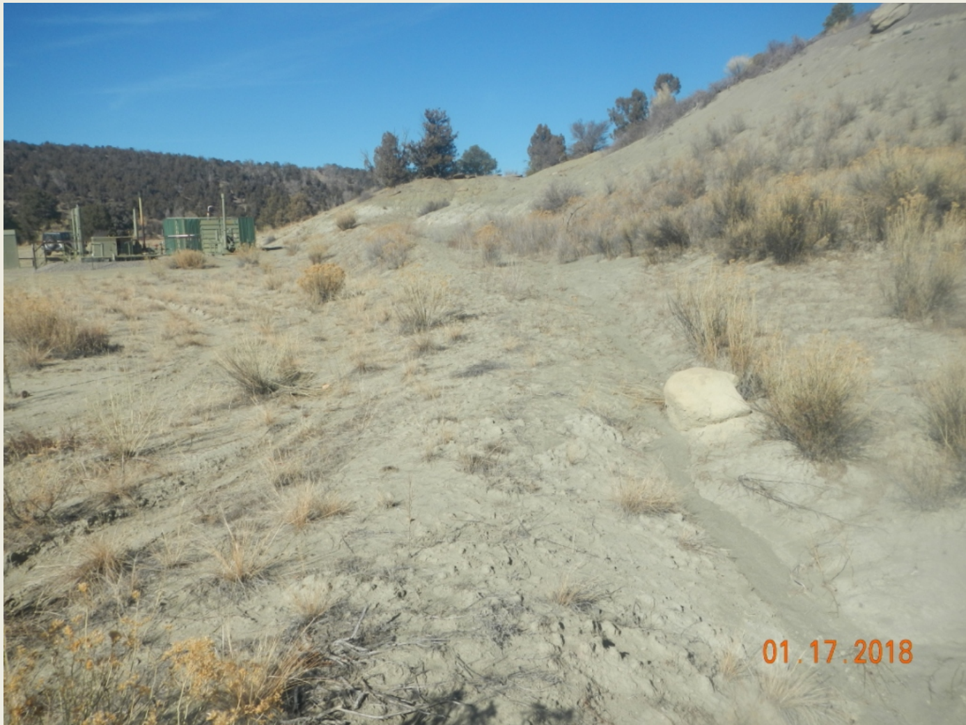
Photo 6. View of diversion channel in northern project area (upstream from photos 5 and 6) that is full of sediment and needs maintenance.
