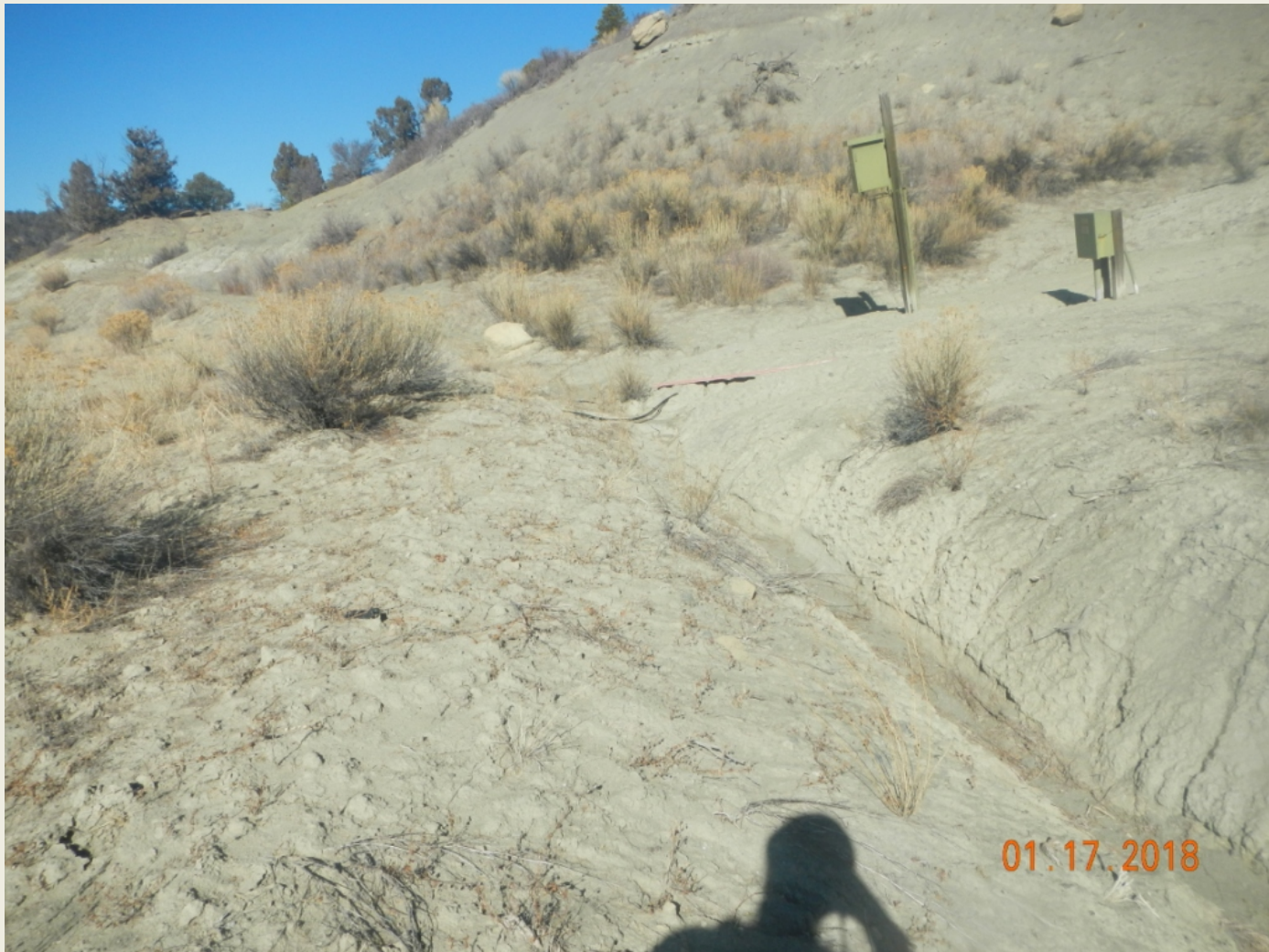
Photo 4. View of diversion channel, approximately 3.5 feet wide and deep, in the northeastern portion of the project area (facing upstream) that is eroding and needs stormwater controls.
