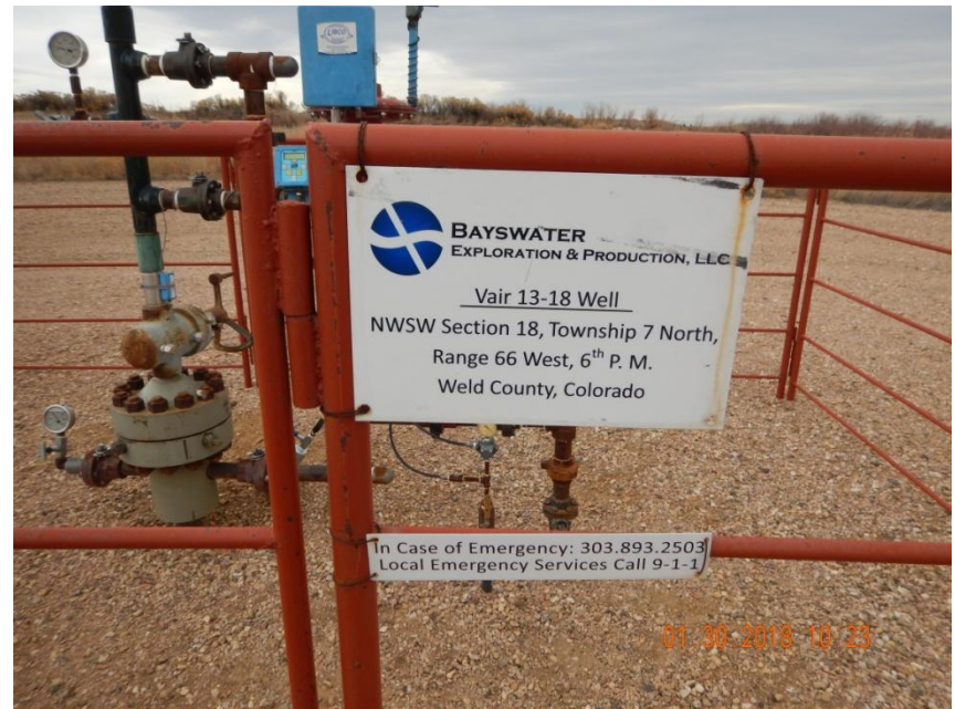
Photo 6. Photo taken of the well head sign at location. The previous Operator sign is not reflective of the current Operator. PDC shall comply with Rule 210.b.
