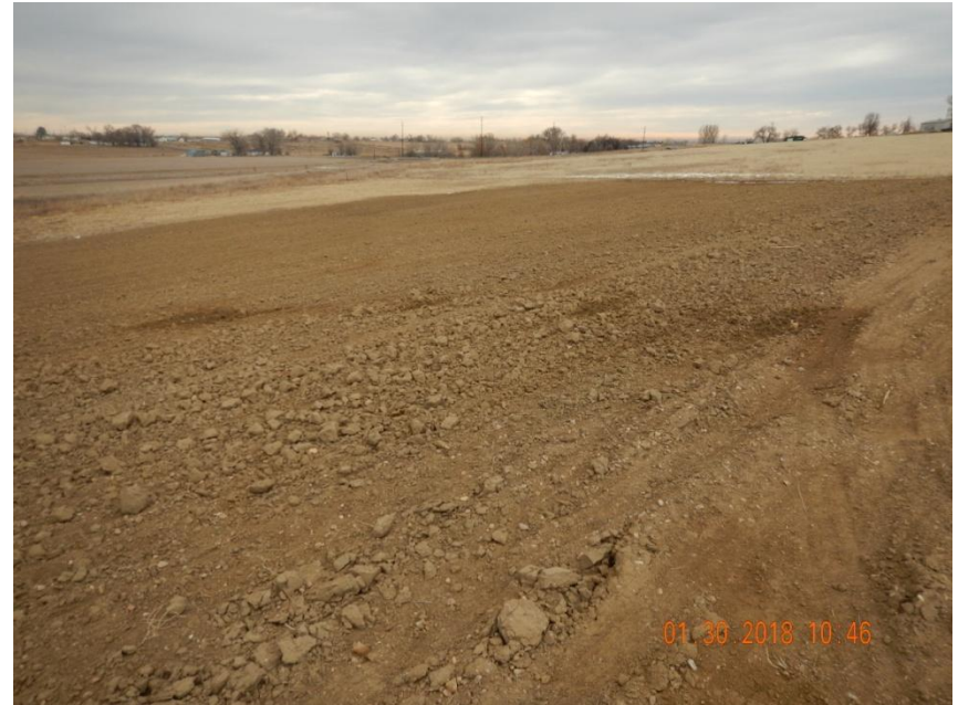
Photo 4. Photo taken from the southeastern location, facing South. See comments under Photo 1. No stormwater BMPs were observed down gradient of the disturbance areas (interim area).
