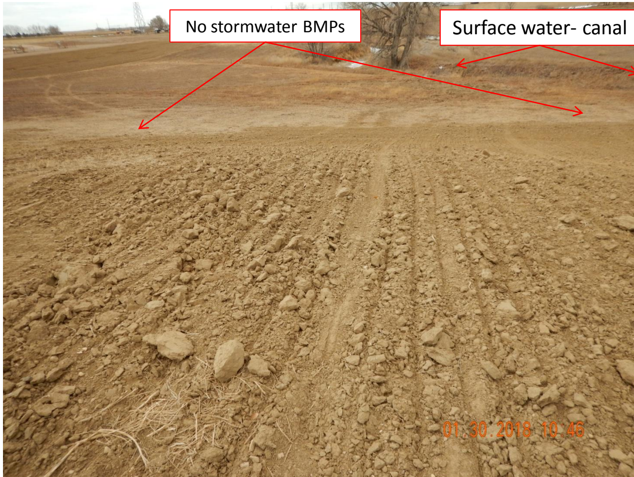
Photo 5. Photo taken from the southeastern location, facing North. See comments under Photo 4. The surface roughening BMP has not been installed in the correct direction. The surface roughening BMP should be installed perpendicular to the slope to help reduce runoff velocity, increases infiltration, and reduces erosion. In this current state, this would aid erosion in a stormwater event.
