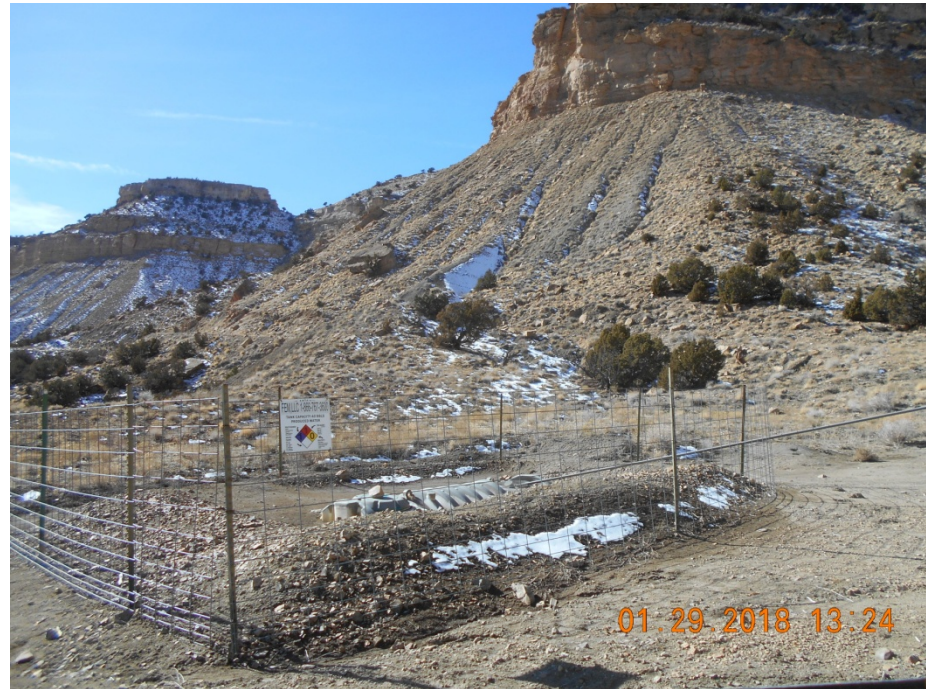
Buried produced water tank looking SW. Note eroded/breached berms on SE corner
