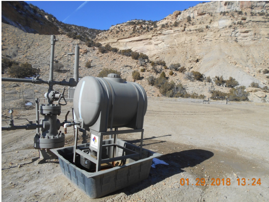
Wellhead and chemical drum with secondary containment.
