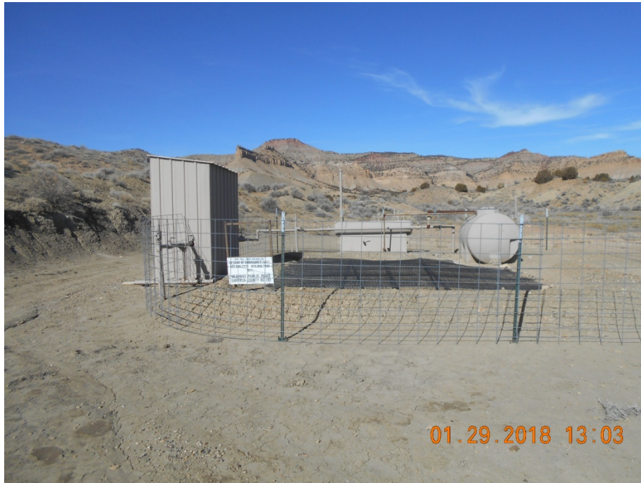
Meter housing, Separator, Tank and Blowdown pit with sign.
