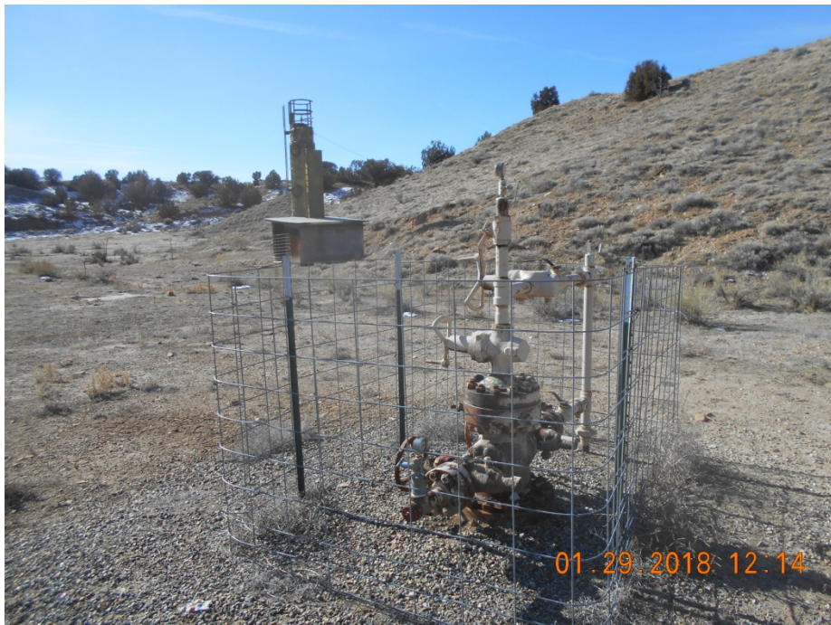
Wellhead looking SW
