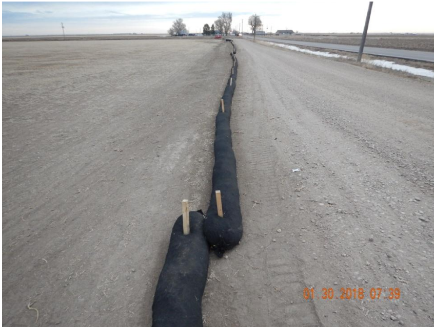
Photo 1. Photo taken from the entrance of location off CR90, facing East. Operator has wattle BMPs throughout the entire access road.
