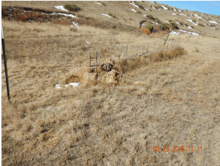
Photo 1: Photo taken from the south end of the location, facing west. Inspection #682502556 required operator to install or repair stormwater and sediment control BMP's on location. Photo shows hay-bale ponding BMP that has not been maintained or repaired, and is not in proper functioning condition. In accordance to good engineering practices, bale and straw wattle BMPs need to be trenched with ends tightly abutted, and backfilled on the up-gradient side and compact. Bales seen here have not been trenched.
