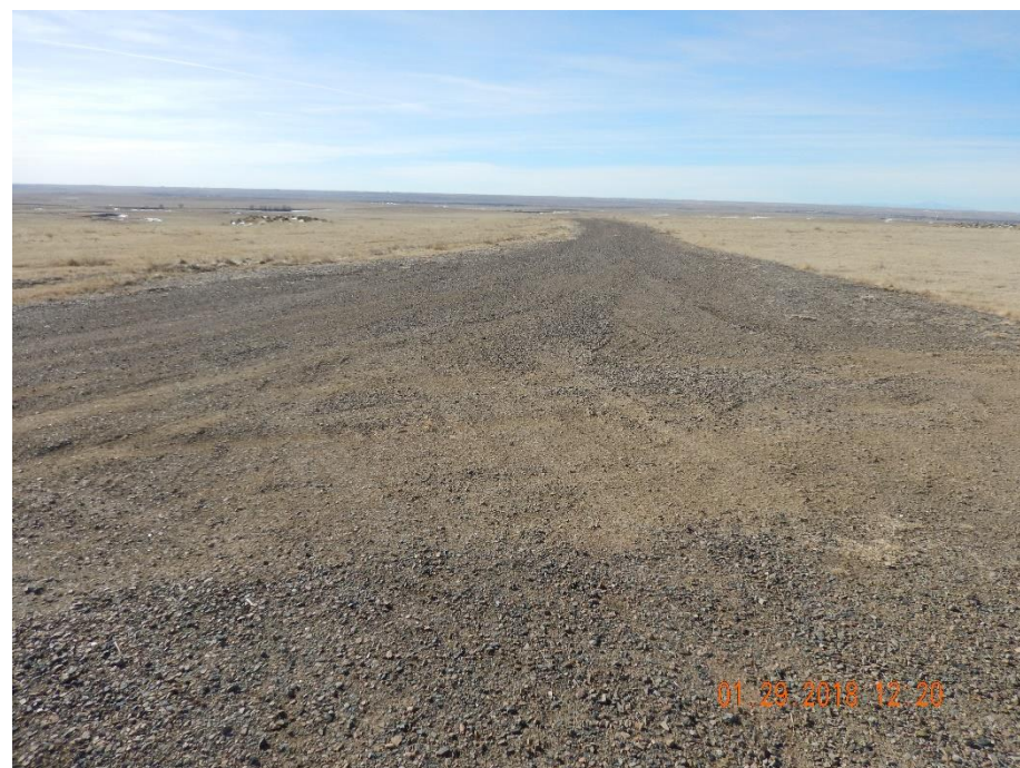
Photo 16: Photo taken from the access road north of the location, facing south. Previous inspections required operator to perform reclamation on the access road. Photo shows access road has not been reclaimed. 6 foot measuring stick for reference.
