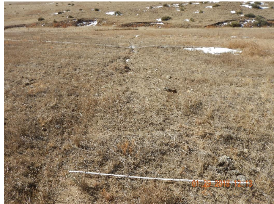
Photo 8 : Photo taken from the southwest end of the location, facing southwest. Photo shows water movement patterns and erosion evident on location.
