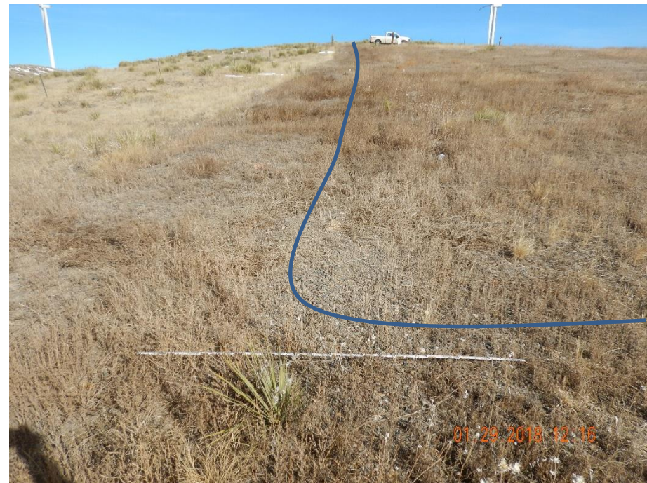
Photo 12: Photo taken from the west end of the location, facing north. Photo shows areas of the access road where road-base and gravel remains. 6 foot measuring stick for reference.
