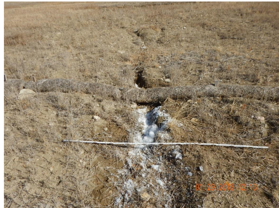
Photo 6: Photo taken from the southwest end of the location. Photo shows straw wattle BMP in not in proper functioning conduction and has not been maintained per corrective actions. Erosion degradation has also not been repaired and stabilized, and has continued to erode since previous inspection. 6 foot measuring stick for reference.
