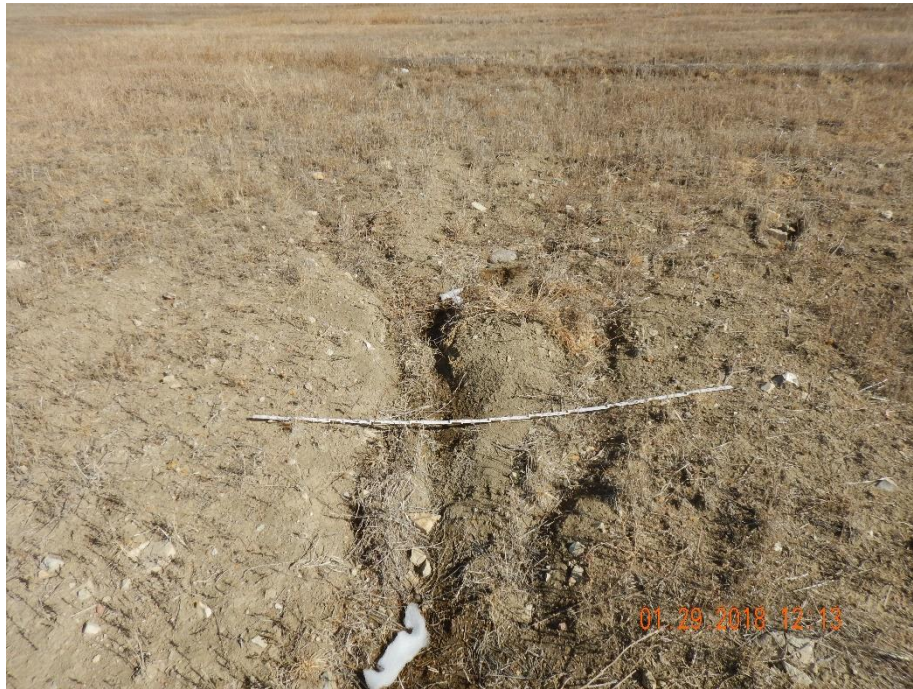
Photo 7: Photo taken from the southwest end of the location, facing north. Photo shows that erosion degradation has not been repaired and stabilized per corrective actions, and has continued to erode since the previous inspection. 6 foot measuring stick for reference.
