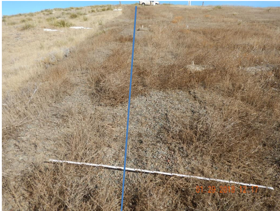
Photo 13: Photo taken from the west end of the location, facing north. Photo shows areas of the access road where road-base and gravel remains. 6 foot measuring stick for reference.
