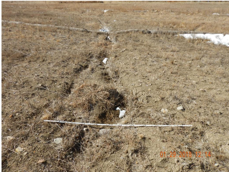
Photo 9: Photo taken from the southwest end of the location, facing southwest. Photo shows that erosion degradation has not been repaired and stabilized per corrective actions, and has continued to erode since the previous inspection. 6 foot measuring stick for reference.
