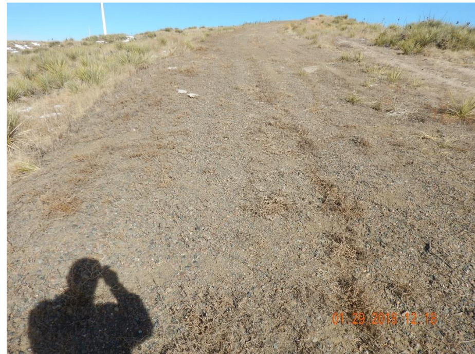
Photo 14: Photo taken from the access road north of the location, facing north. Previous inspections required operator to perform reclamation on the access road. Photo shows access road has not been reclaimed. 6 foot measuring stick for reference.
