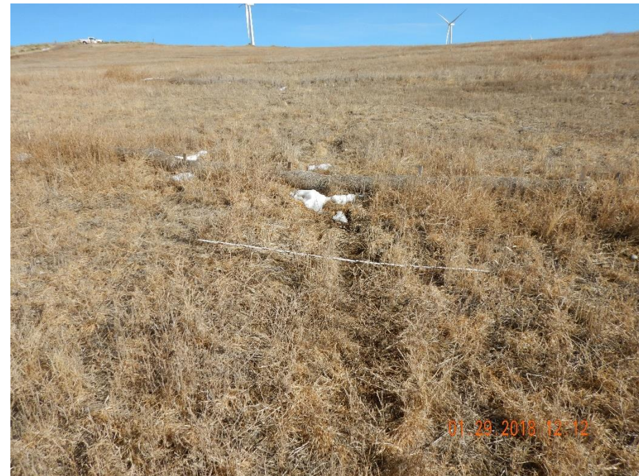
Photo 4: Photo taken from the southwest end of the location, facing north. Photo shows erosion remains evident, and stormwater and sediment control BMP has not been maintained per corrective actions. Stormwater has continued to cut under the wattle with additional degradation since previous inspection evident. 6 foot measuring stick for reference.
