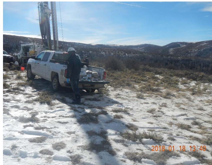
On location of MW-22
