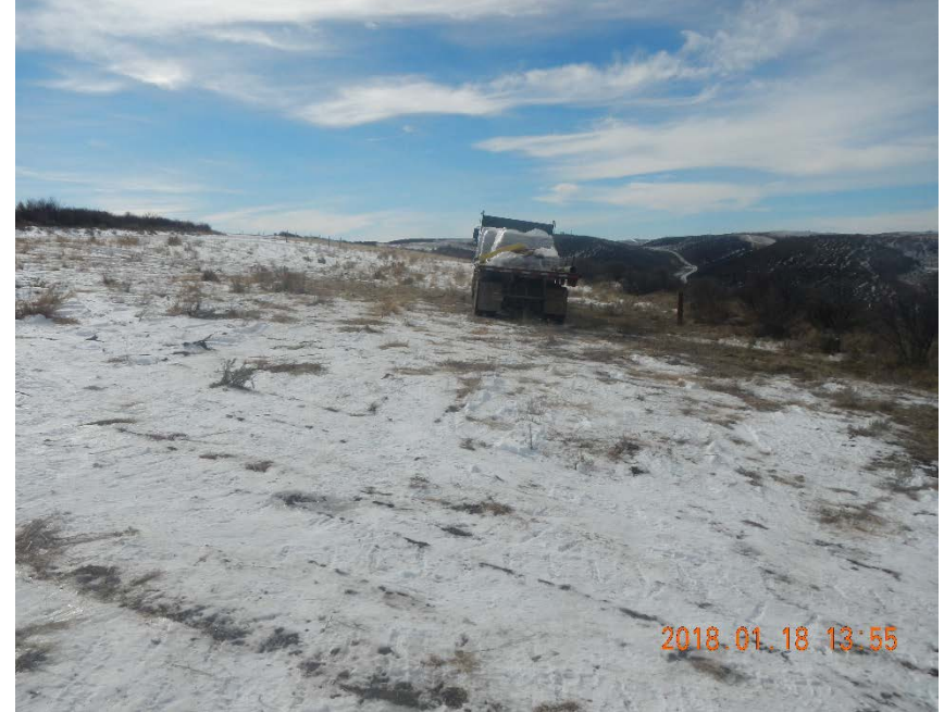
MW-21. Located on the right-of-way on Divide Rd. at approximately 200 ft east of the release point. Caerus personnel reported that a sheen had been observed in this well.
