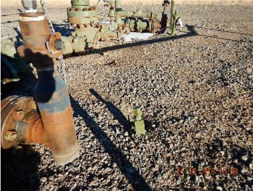
Photo 3: Unused 1" steel riser at wellhead.
