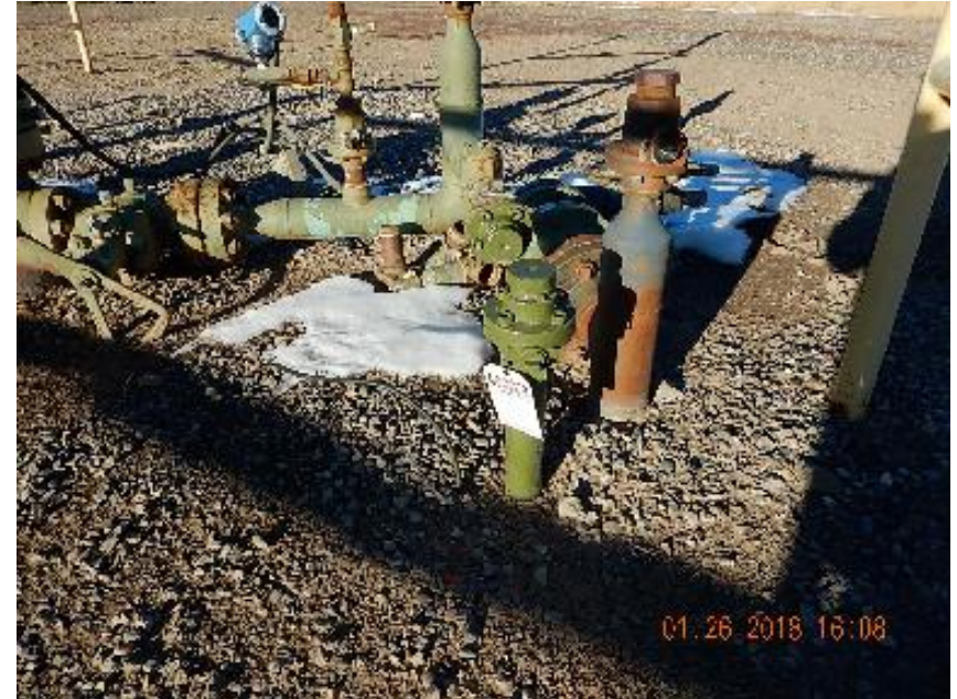
Photo 2: Unused plugged and tagged 2" steel riser at wellhead.
