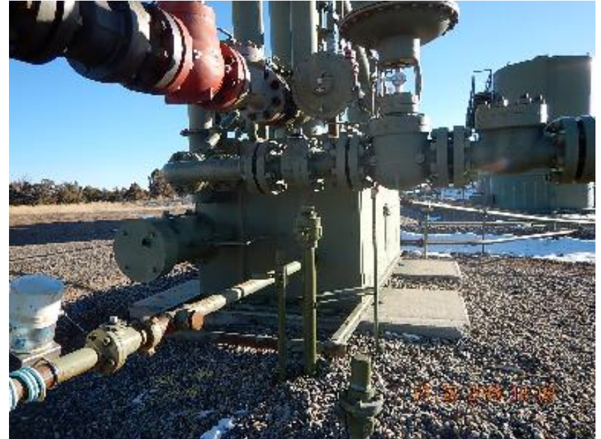
Photo 4: Unused (2) 2" and 1" steel risers at separator.
