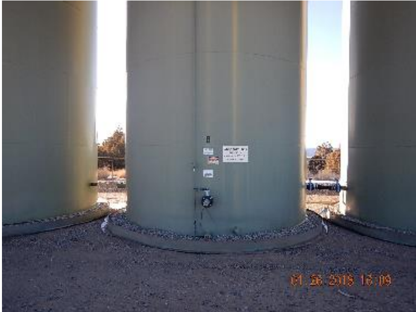
Photo 5: Labels on production tank. Picture taken from top rail of fence. The top label in the row of three is the NFPA label.
