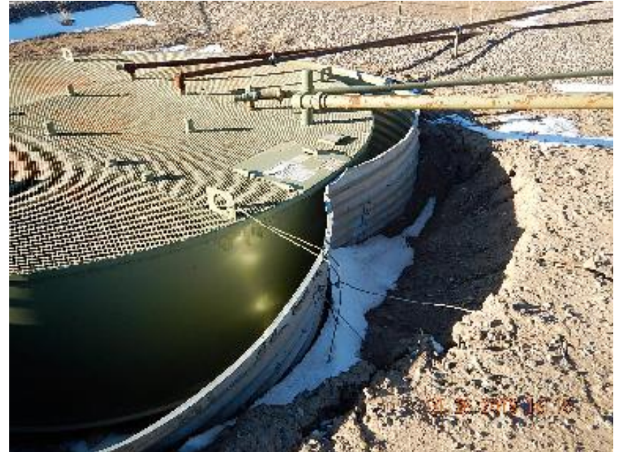
Photo 6: Collapsed containment wall on E side of open top tank.
