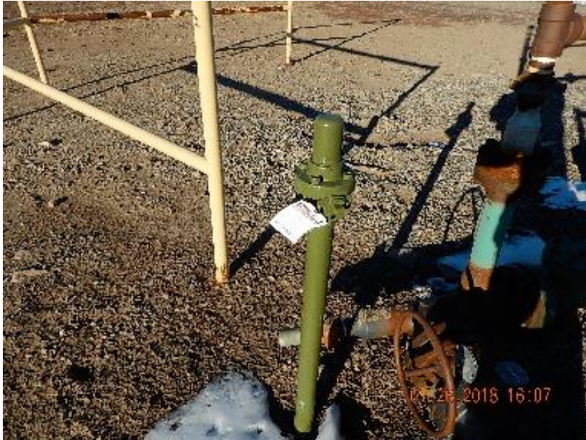
Photo 1: Unused plugged and tagged 2" steel riser at wellhead.
