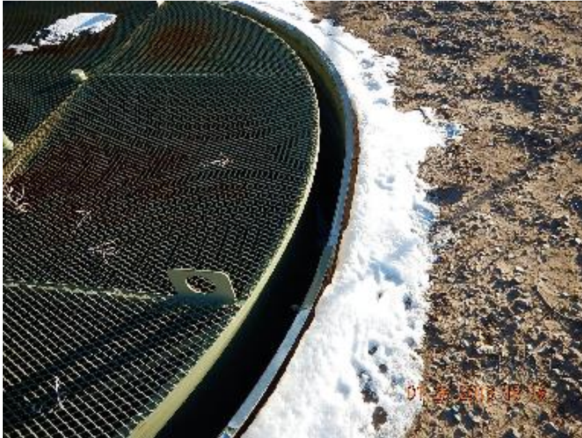
Photo 7: Tank pushed to the W side of containment wall.
