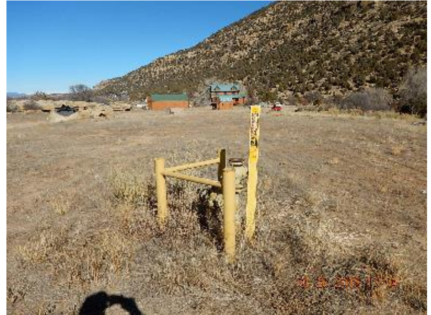
Photo 8: E side riser with steel post and pole barrier.
