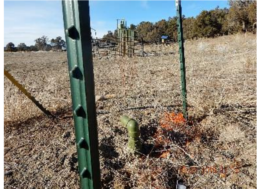
Photo 2: Unused steel riser.
