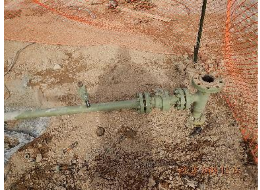
Photo 4: Riser at wellhead.
