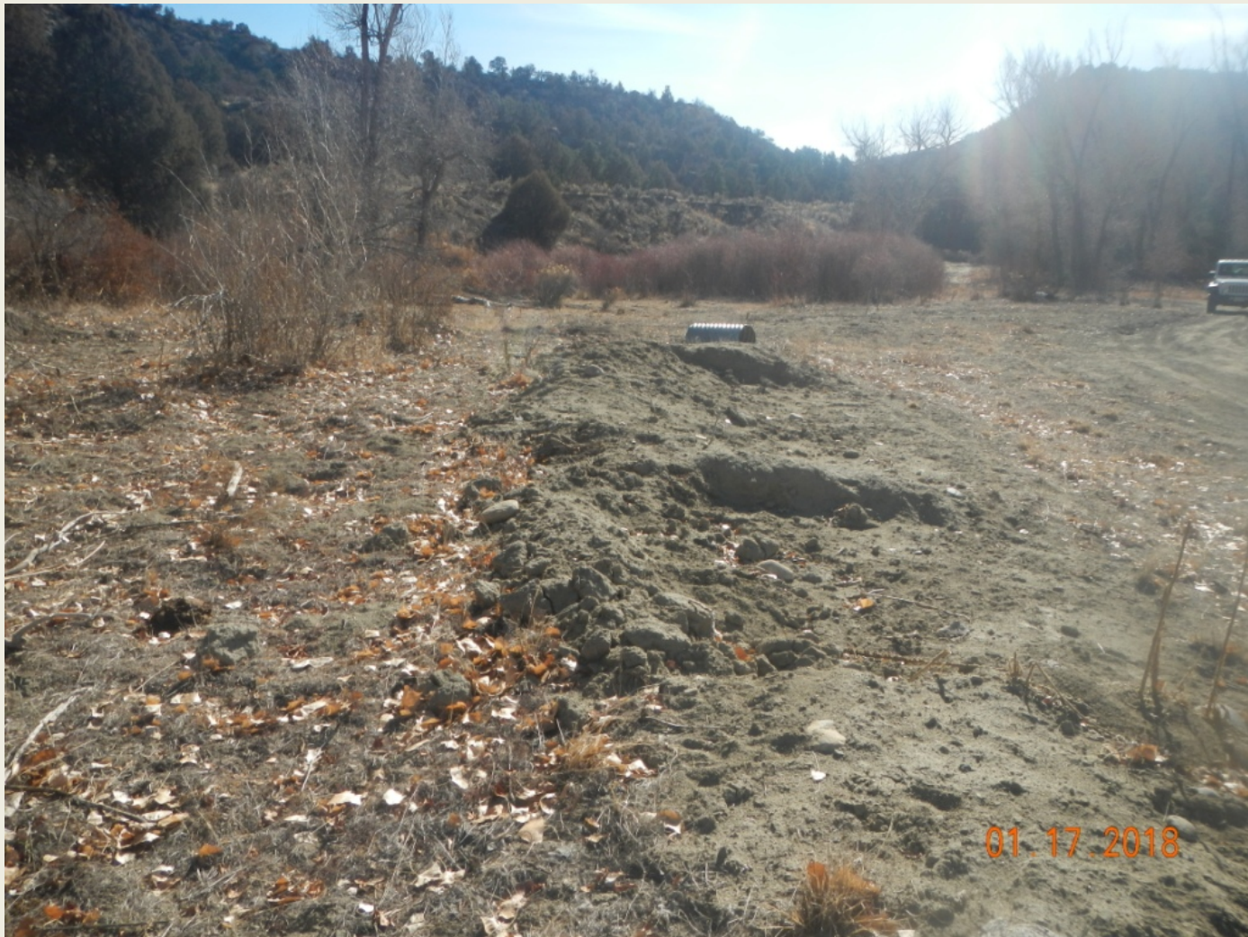
Photo 4. View sediment piles in the eastern portion of the project area. Sediment needs to be contained to prevent run-off and run-on.
