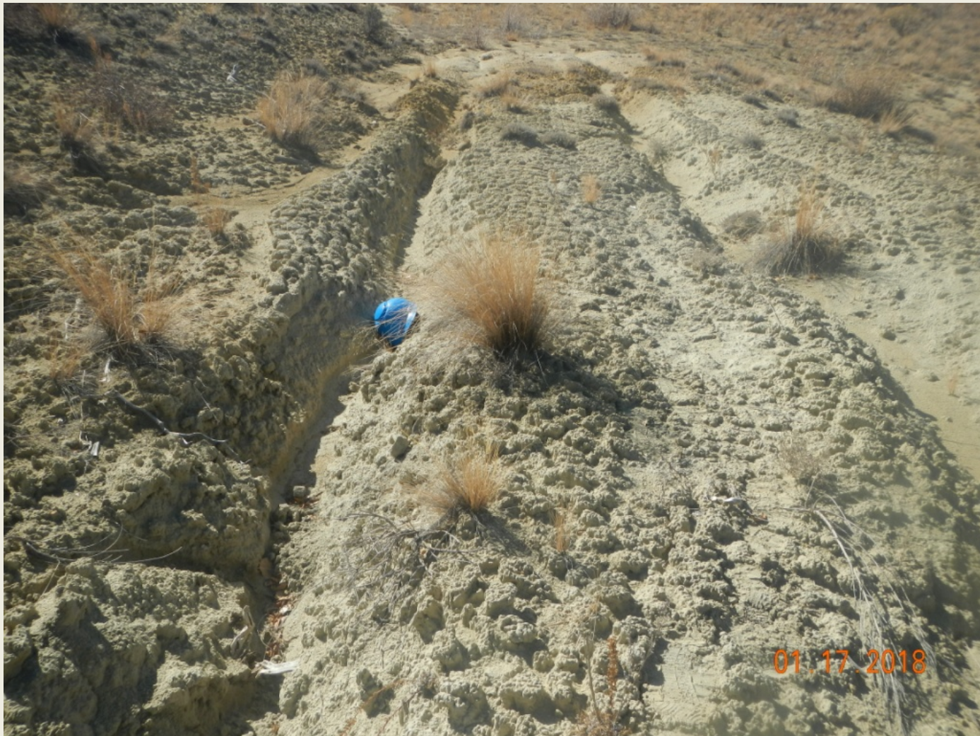
Photo 4. View of erosional pedestaling and channeling (approximately 1.5 feet wide and deep) within the access road.
