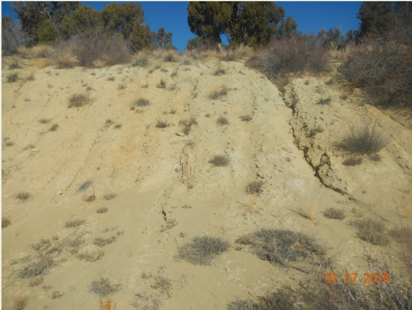
Photo 9. View of erosional channels forming within the northern cut-slope.
