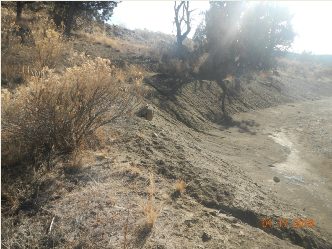
Photo 4. View of area in the northeastern corner of the well pad where stormwater flows run-onto the well pad and are eroding the cut-slope. Diversion ditches are full of sediment.
