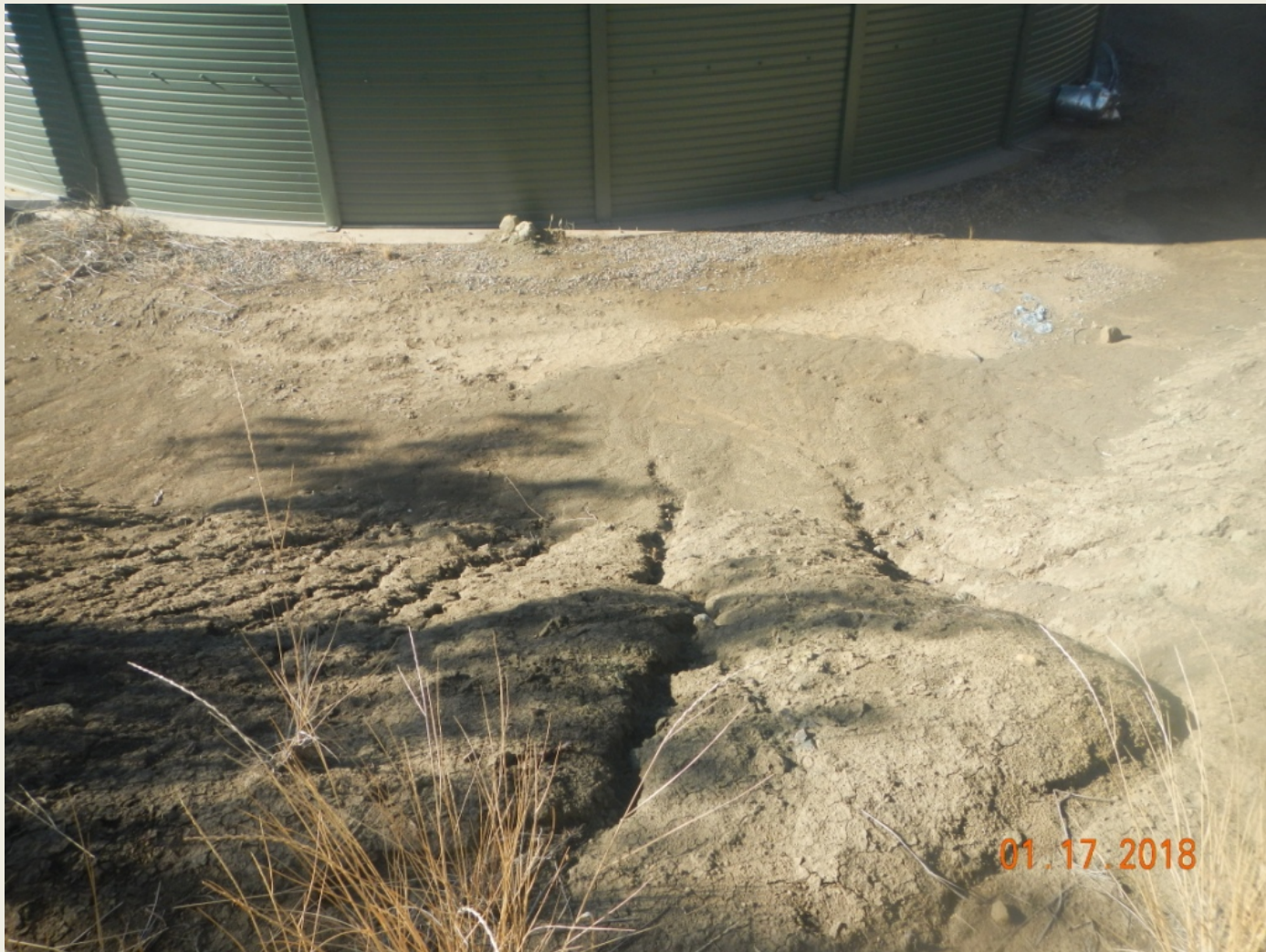
Photo 5. View of sediment deposition and erosional channeling in the northeastern portion of the project area.
