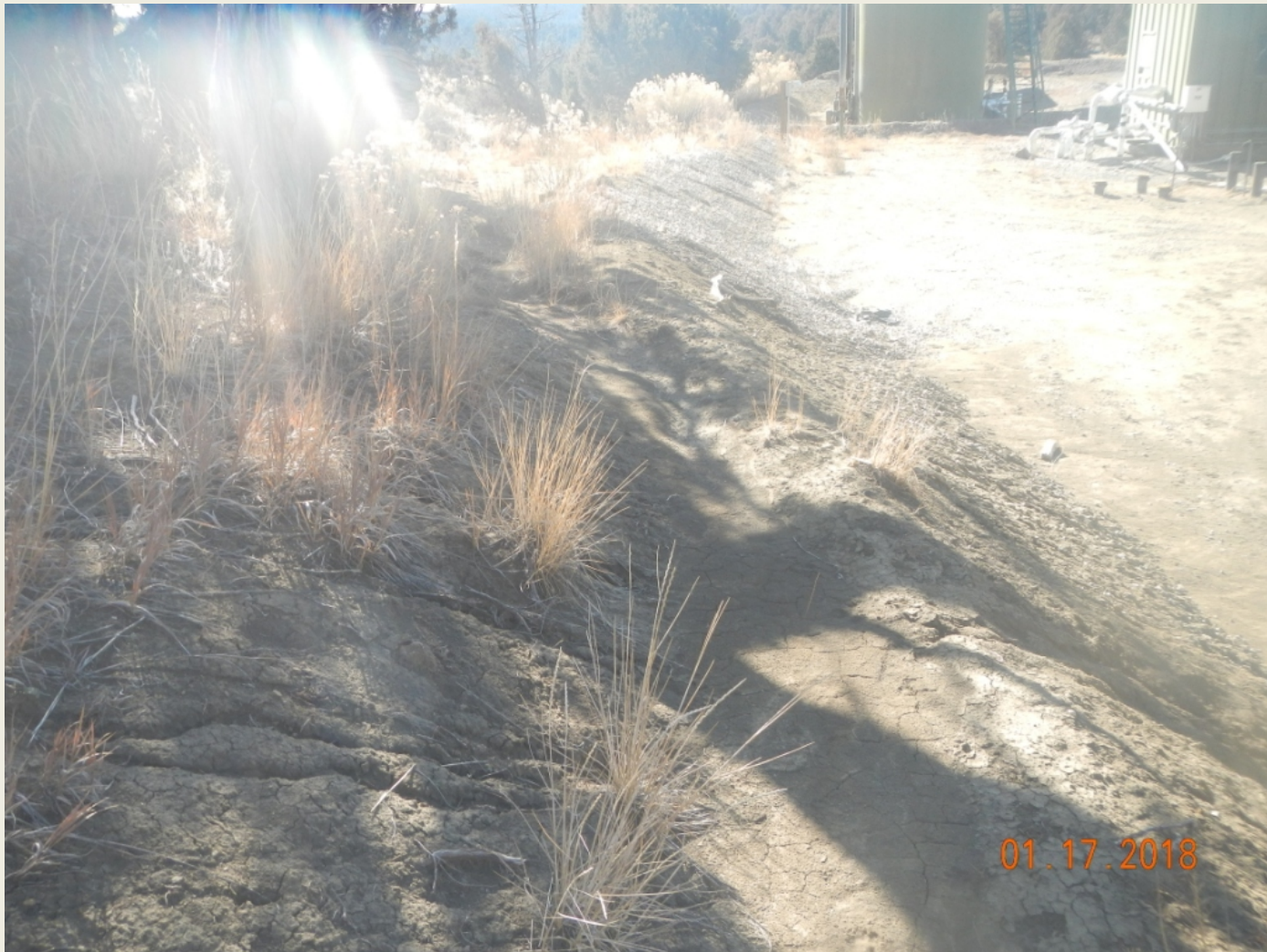
Photo 6. Another view of erosional channeling and diversion full of sediment in the northeastern corner of the project area.
