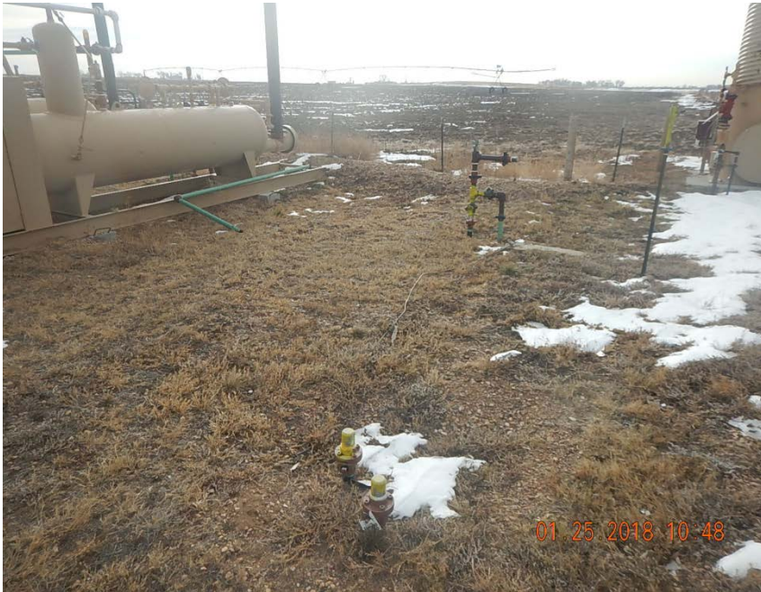
Photo 5: Marked, tagged risers W of separators
