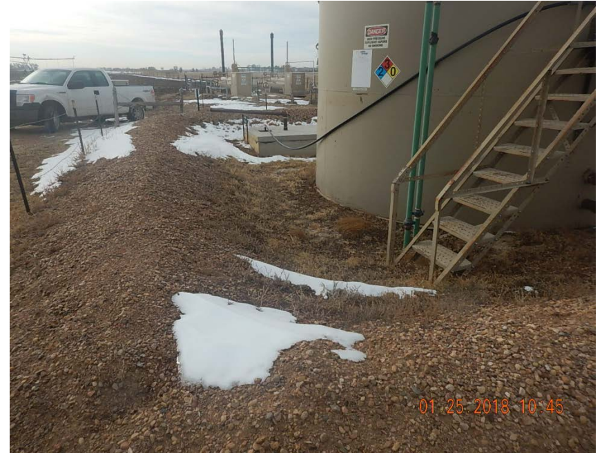
Photo 4: Weeds in tank battery, berm
