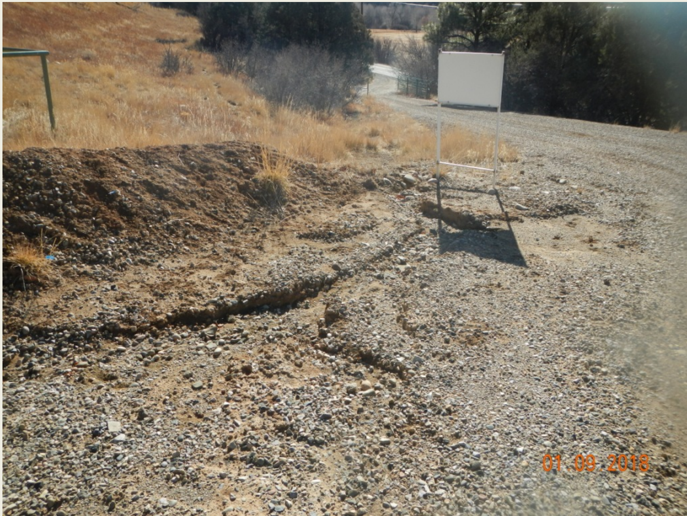
Photo 5. View of erosion occurring at the well pad entrance facing southward.
