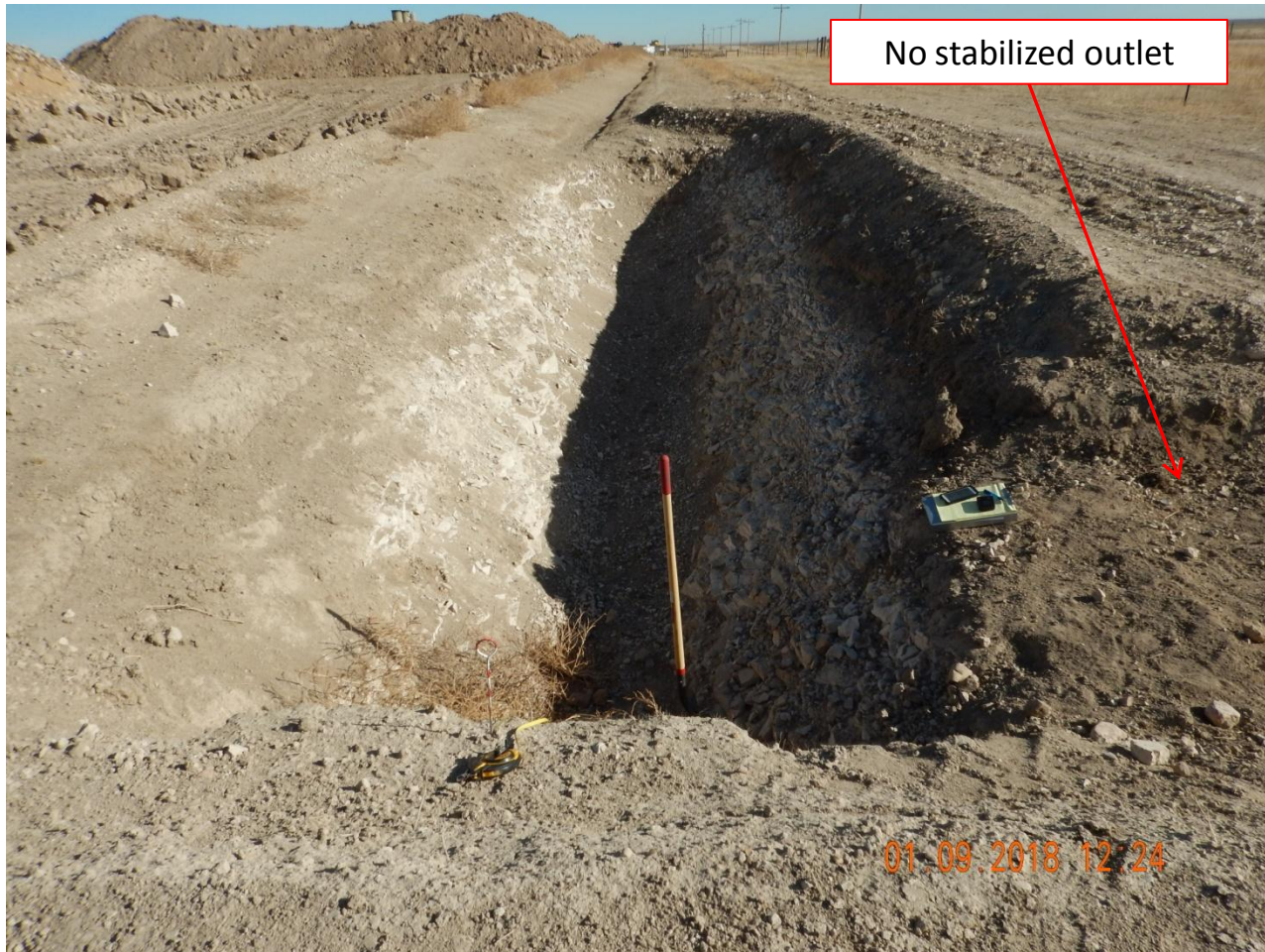
Photo 3. Photo taken from sediment trap #1, facing East. Operator has installed the above sediment trap since the previous inspection. Rock material from the sediment trap has been removed; therefore, the sediment trap has no stabilized outlet. Interim reclamation activities were occurring during the time of the inspection but stormwater BMPs were not maintained. Also, this does not appear to be built to Noble's own Stormwater BMP Manual (i.e., side slopes not 2:1) or in accordance with good engineering practices.
