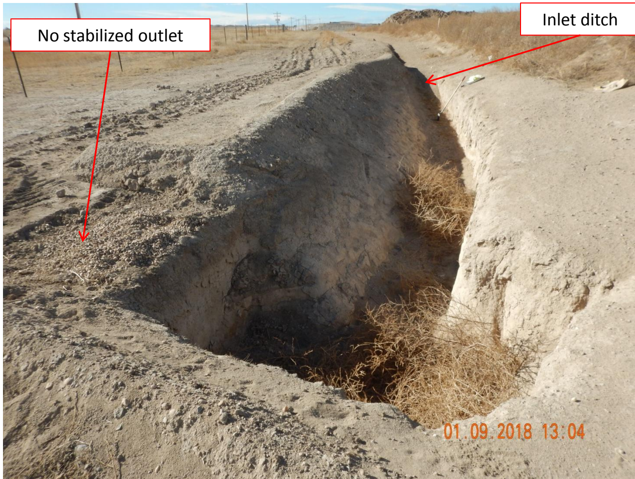
Photo 4. Photo taken from 'sediment trap' #2, facing West. Operator has enlarged the above 'sediment trap' since the previous inspection; however, it is not constructed properly. The outlet area appears to be higher than the inlet ditch and the outlet rock material has been removed. Based on the above description, this would not be considered a constructed sediment trap. This would be considered an enlarged ditch with no stabilized outlet. Photo also indicates unmanaged weed debris on location.
