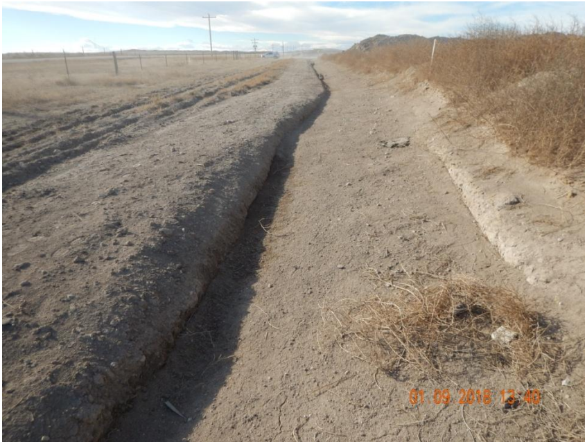
Photo 5. Photo taken from the southeast perimeter of the Earp Pad, facing West. Ditch BMP appears to be filled from wind erosion sediment deposition. Ditch BMP has not been properly installed and does not appear to be installed to Noble's own Stormwater BMP Manual (i.e., not parabolic ditch). Photo also indicates unmanaged weed debris on location.
