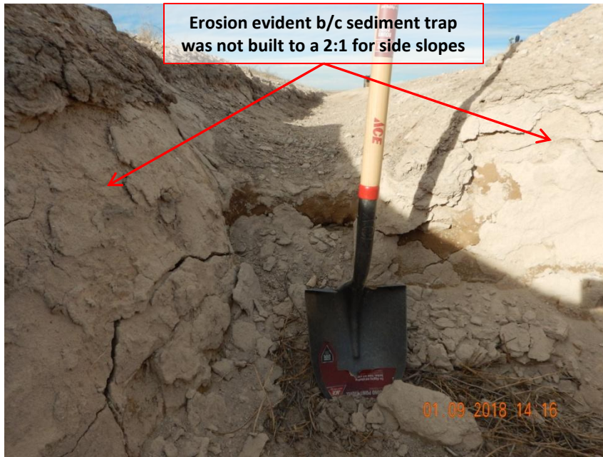
Photo 12. Photo taken from the ditch inlet area of 'sediment trap' #5, facing East. Inlet ditch is approximately 1.5' in height. Shovel is at the bottom of the 'sediment trap' area which was used to measure the height of the inlet.
