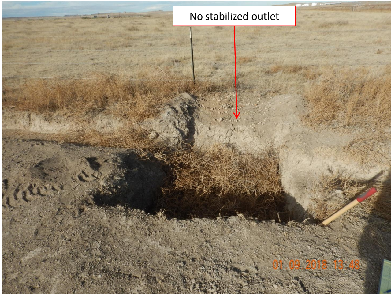
Photo 8. Photo taken from 'sediment trap' #4, facing North. See comments under Photo 4- all comments apply to this 'sediment trap' and weed debris. See photos 9 & 10 to further illustrate how the sediment trap has not been constructed properly.
