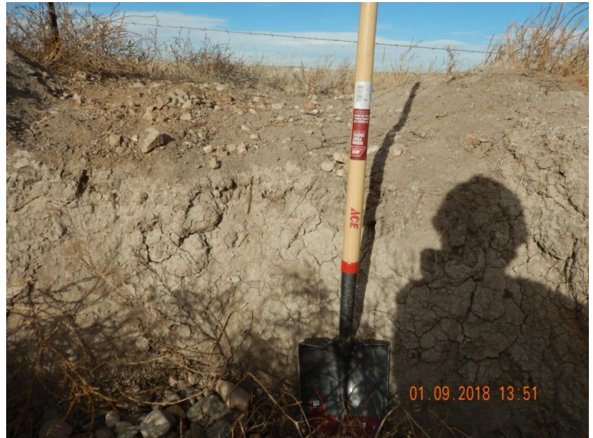
Photo 10. Photo taken from the outlet area of 'sediment trap' #4, facing North. Outlet is approximately 3' in height which is higher than the inlet ditch; therefore, this would not function as a sediment trap. Shovel is at the bottom of the 'sediment trap' area which was used to measure the height of the outlet.
