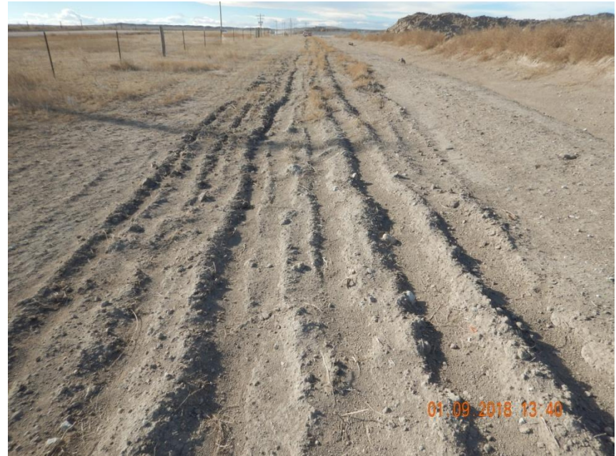
Photo 6. Photo taken from the southeast perimeter of the Earp Pad, facing West. Surface roughening BMP in need of maintenance, as it appears to be filled from wind erosion sediment deposition. Photo also indicates unmanaged weed debris on location.
