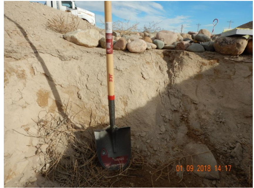
Photo 13. Photo taken from the outlet area of 'sediment trap' #5, facing North. The outlet is approximately 2.5' in height which is higher than the inlet ditch; therefore, this would not properly function as a sediment trap. Shovel is at the bottom of the 'sediment trap' area which was used to measure the height of the outlet.
