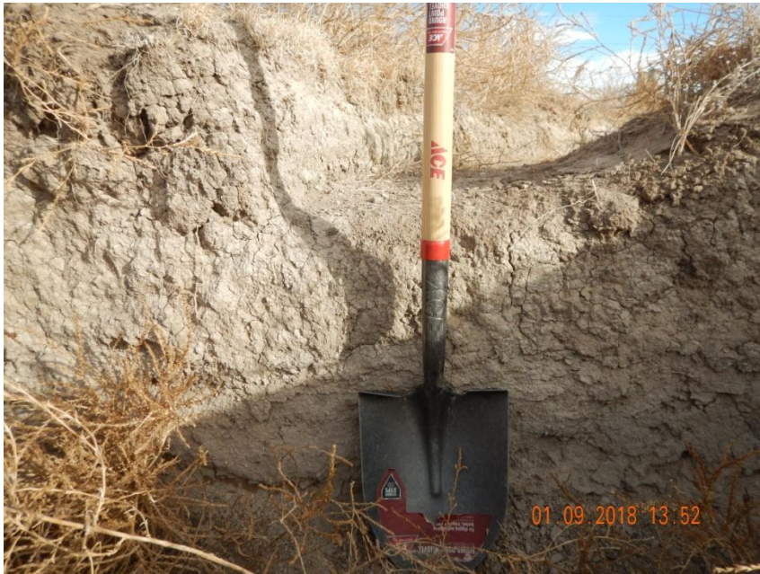
Photo 9. Photo taken from the ditch inlet area of 'sediment trap' #4, facing East. Inlet ditch is approximately 2' in height. Shovel is at the bottom of the 'sediment trap' area which was used to measure the height of the inlet.
