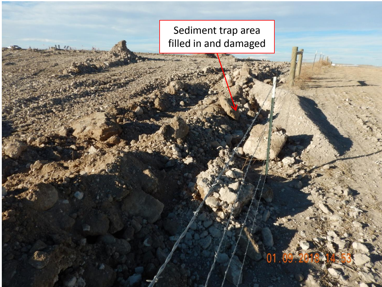
Photo 21. Photo taken from sediment trap #9, facing North. Stormwater controls have been removed- see comments under Photo 18.
