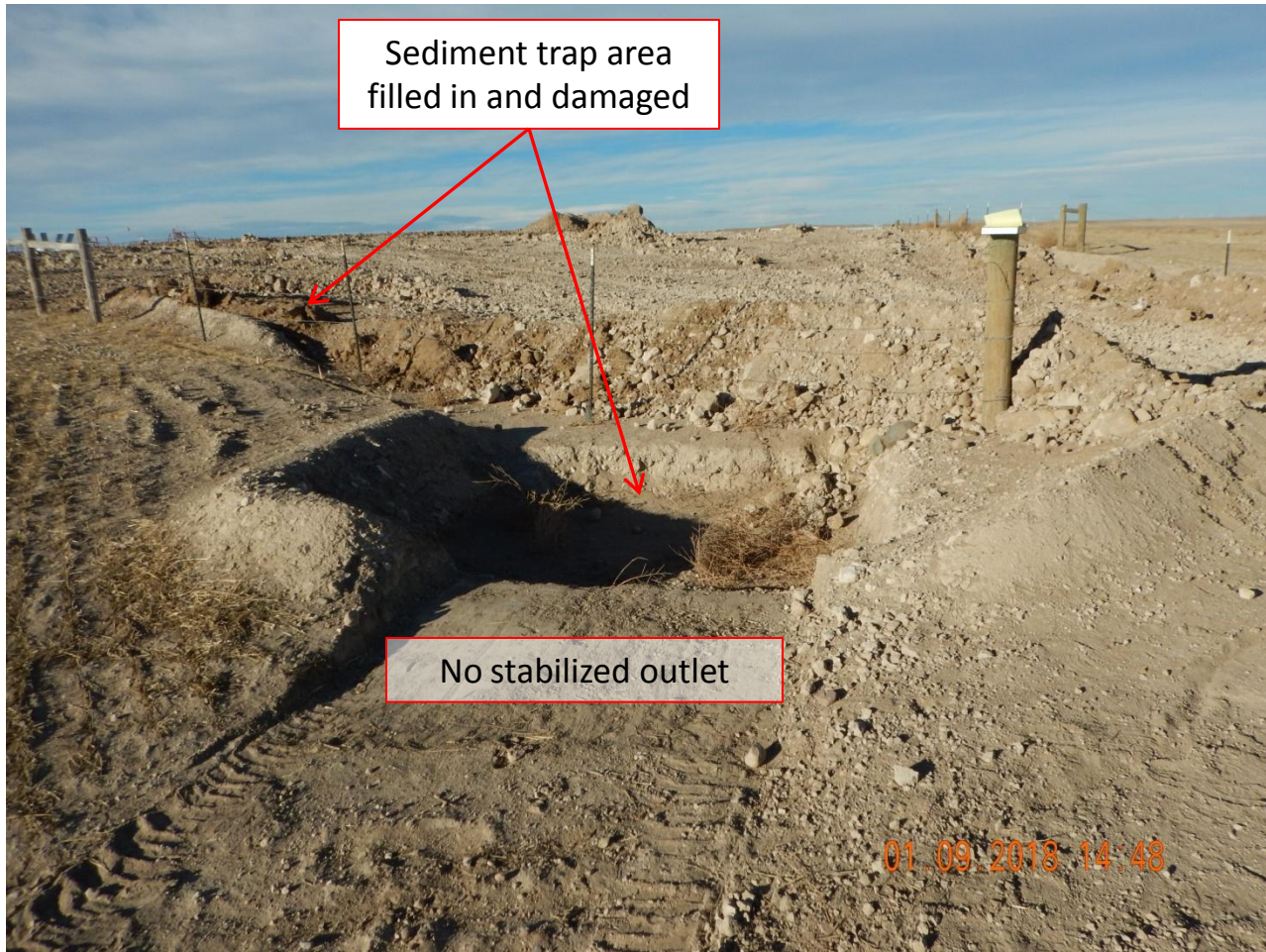
Photo 19. Photo taken from sediment trap #8, facing North. Stormwater controls have been removed- see comments under Photos 18.
