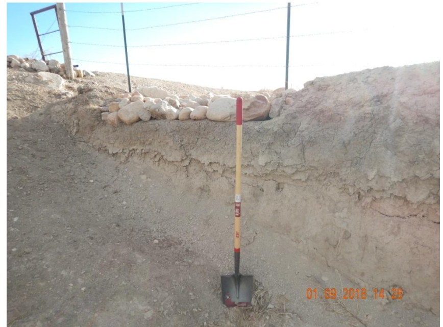
Photo 16. Photo taken from the outlet area of 'sediment trap' #6, facing South. The outlet is approximately 4.5' in height which is higher than the inlet ditch; therefore, this would not properly function as a sediment trap. Shovel is at the bottom of the 'sediment trap' area which was used to measure the height of the outlet.
