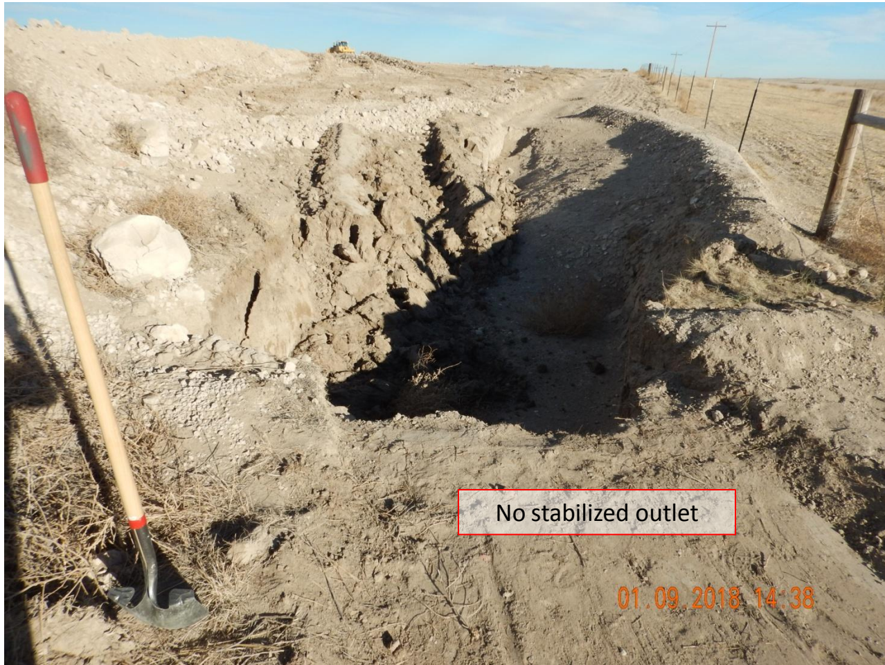
Photo 18. Photo taken from sediment trap #7, facing East. Stormwater BMP has been damaged and not functional. Rock material from the sediment trap has been removed; therefore, the sediment trap has no stabilized outlet. Interim reclamation activities were occurring during the time of the inspection but stormwater BMPs were either removed or not maintained.
