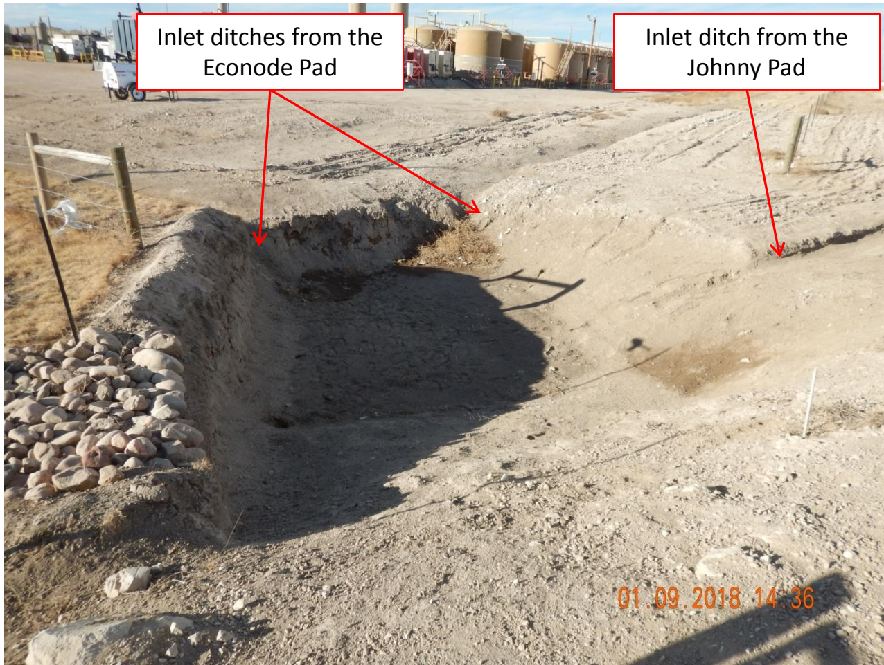
Photo 17. Photo taken from 'sediment trap' #6, facing North. Photo illustrates this 'sediment trap' is being shared with the adjacent Johnny Pad to the east. Ditch BMPs have not been properly installed and does not appear to be installed to Noble's own Stormwater BMP Manual (i.e., not parabolic ditch).
