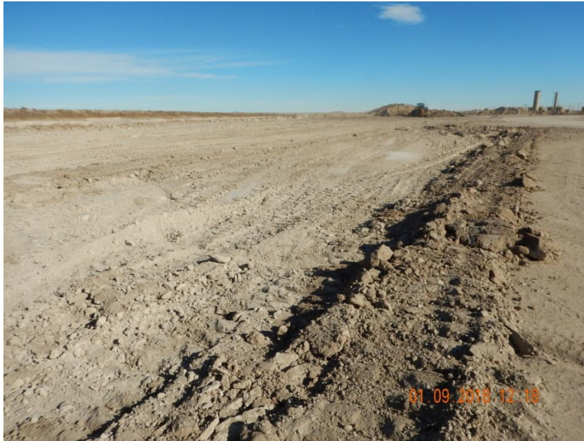
Photo 1. Photo taken from the northwest Earp Pad, facing East. Operator in-process of performing interim reclamation activities. Stormwater BMPs were not maintained or in some cases did not exist during interim reclamation activities.
