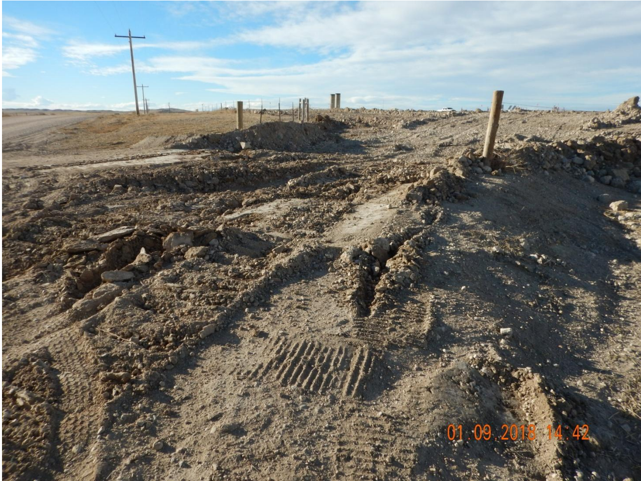
Photo 20. Photo taken from the eastern entrance to the Johnny Pad, facing Northwest. No stormwater BMPs installed around this area during interim reclamation activities.
