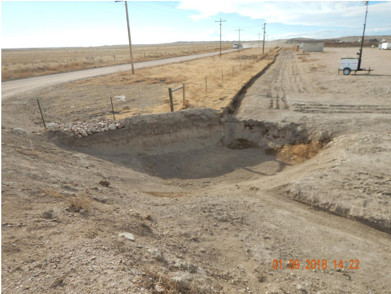
Photo 14. Photo taken from 'sediment trap' #6, facing West. See comments under Photo 4- all comments apply to this 'sediment trap'. See comments under Photo 11 for outlet material. The above outlet has not been constructed using good engineering practices. See photos 15 & 16 to further illustrate how the 'sediment trap' has not been constructed properly.
