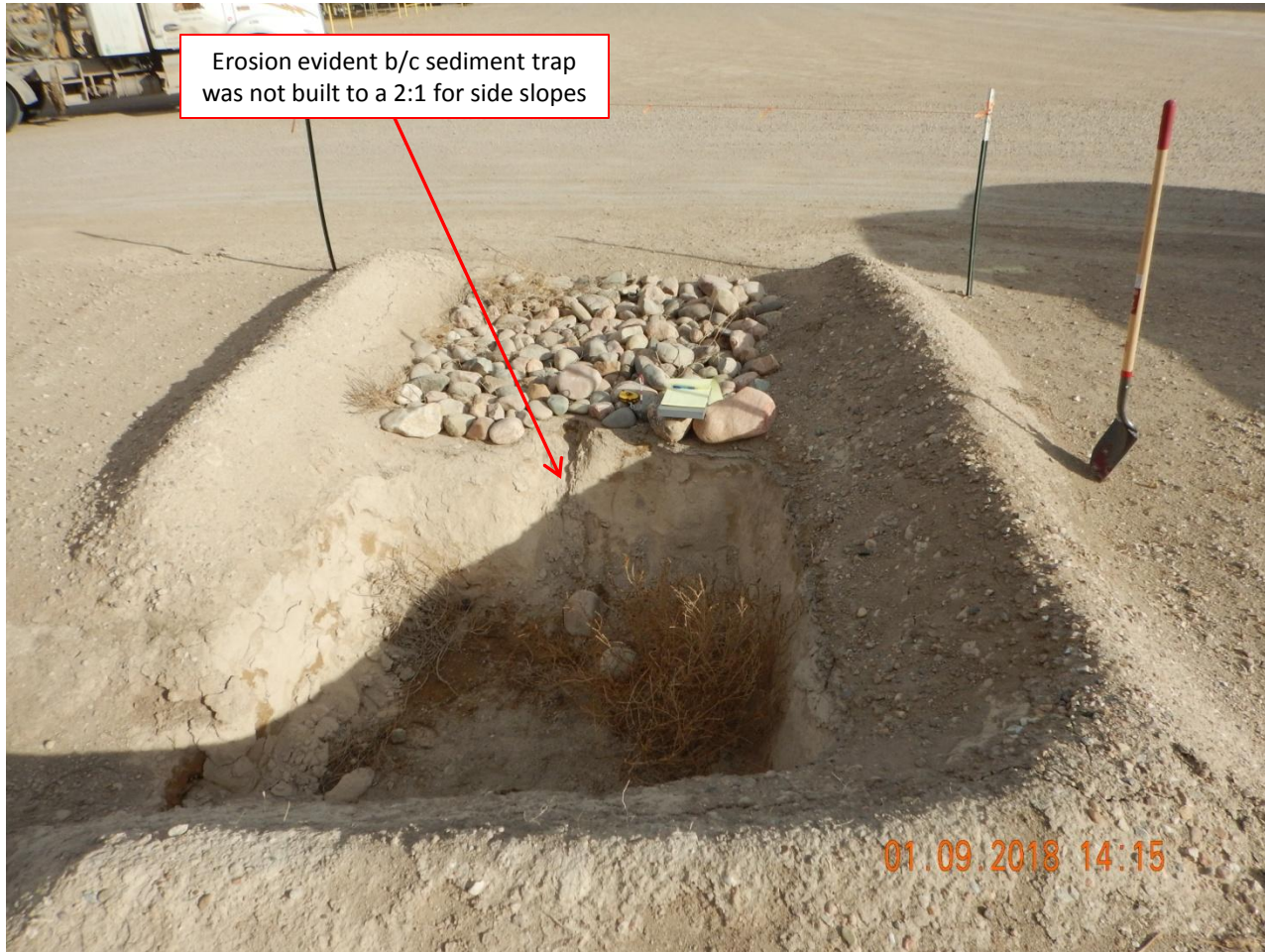
Photo 11. Photo taken from 'sediment trap' #5, facing East. See comments under Photo 4- all comments apply to this 'sediment trap'. Outlet material per good engineering practices should be a combination of coarse aggregate and angular rip rap. The above outlet has not been constructed in accordance with good engineering practices. If it was to discharge from the outlet, it would discharge back onto location which could cause other stormwater issues, for example ponding and vehicle tracking. See photos 12 & 13 to further illustrate how the 'sediment trap' has not been constructed properly.
