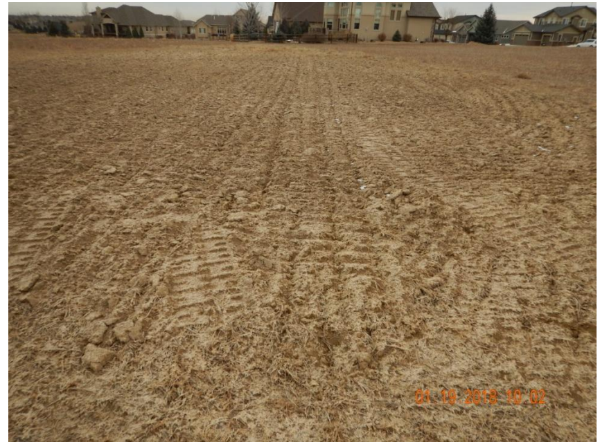
Photo 2. Photo taken from the western location on January 19, 2018, facing East. Operator has performed final reclamation activities. Location has been temporarily stabilized with mulch.
