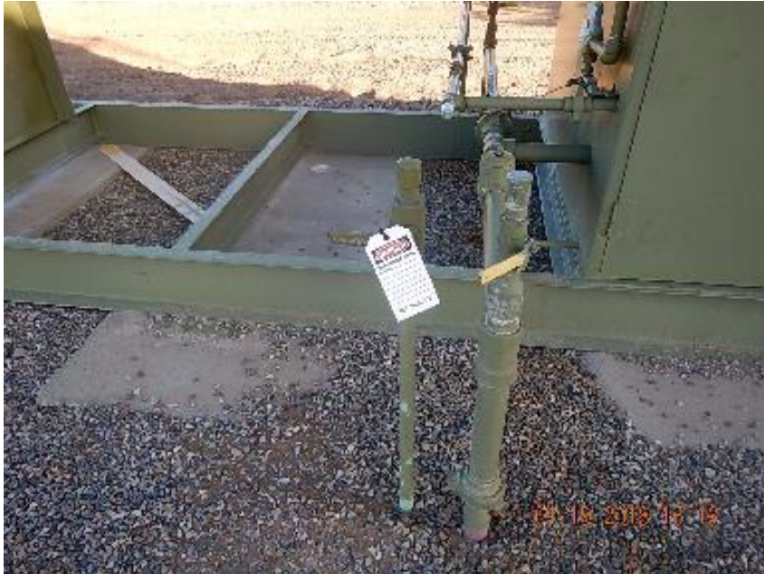
Photo 3: Plugged and tagged 1" steel riser at separator.
