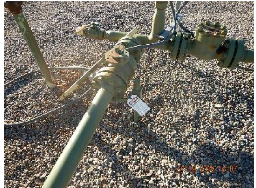
Photo 2: Plugged and tagged 1" steel riser at wellhead.
