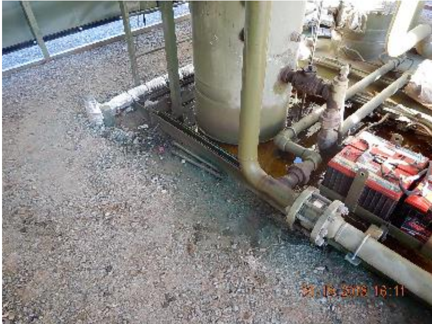
Photo 5: Impacted soil inside compressor carport at knock out pot.
