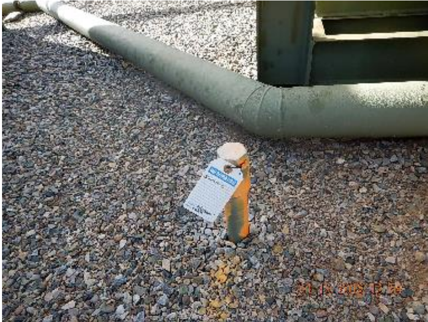
Photo 3: Painted, plugged, and tagged steel riser at separator.
