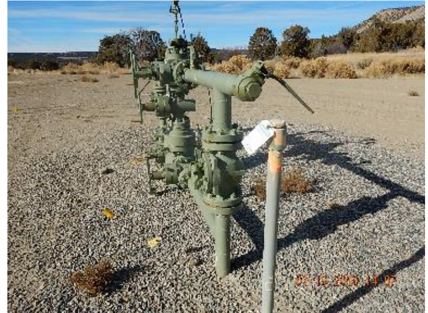
Photo 4: Painted, plugged, and tagged steel riser at wellhead.
