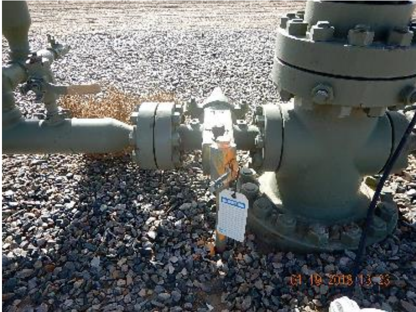
Photo 3: Painted, plugged, and tagged 1" steel riser.
