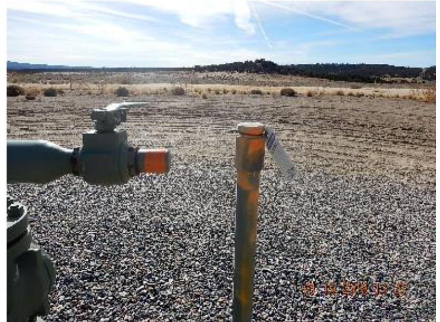
Photo 4: Painted, plugged, and tagged 3" steel riser.
