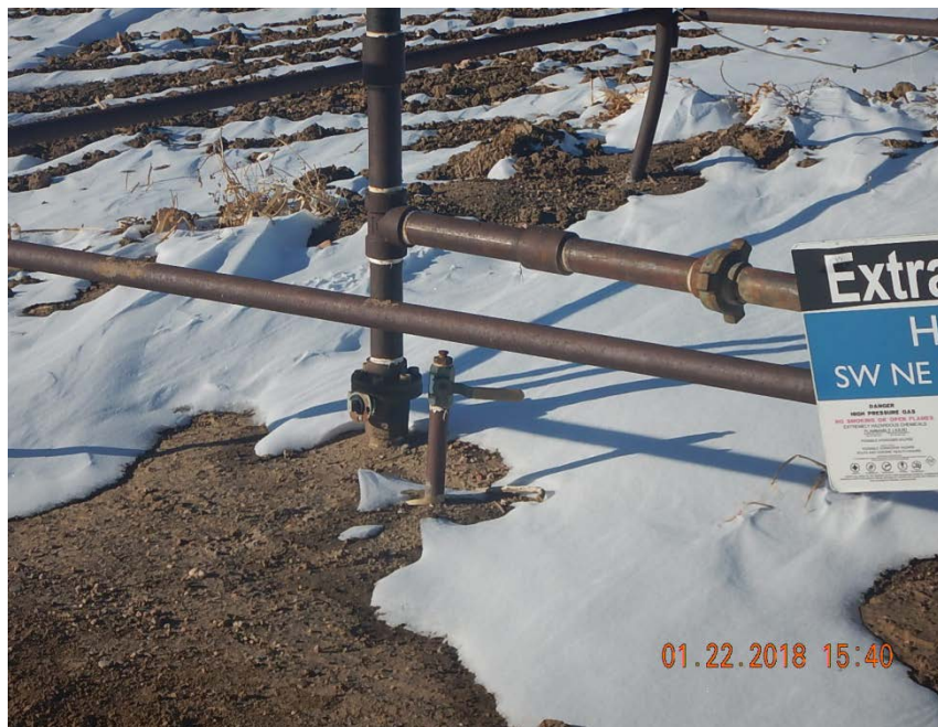
Photo 3: Riser at wellhead
