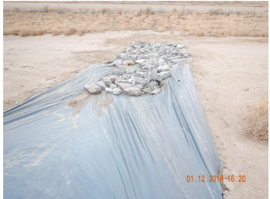
Photo 2. Photo taken from the eastern location, facing East. Unconsolidated soil material along the eastern fill slope. Operator needs to stabilize all unconsolidated soil material.
