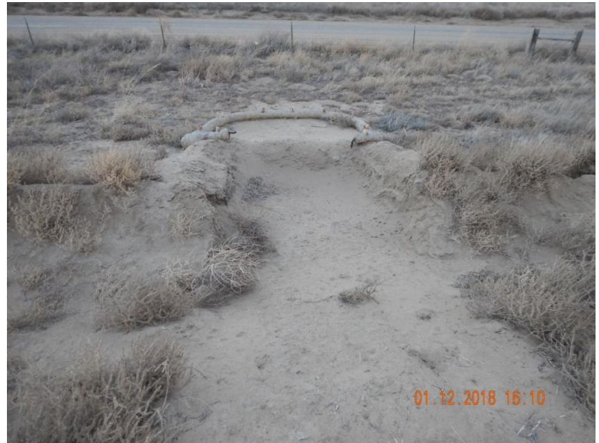
Photo 2. Photo taken from the eastern location, facing East. Sediment trap in need of maintenance- sediment accumulation.
