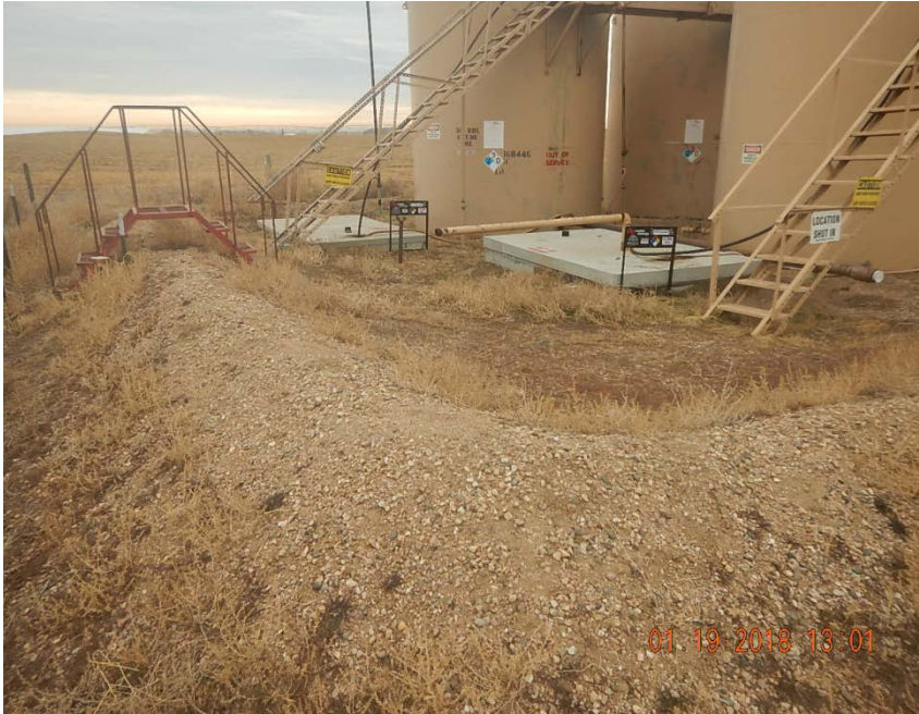
Photo 3: Weeds in tank battery, growing on berms
