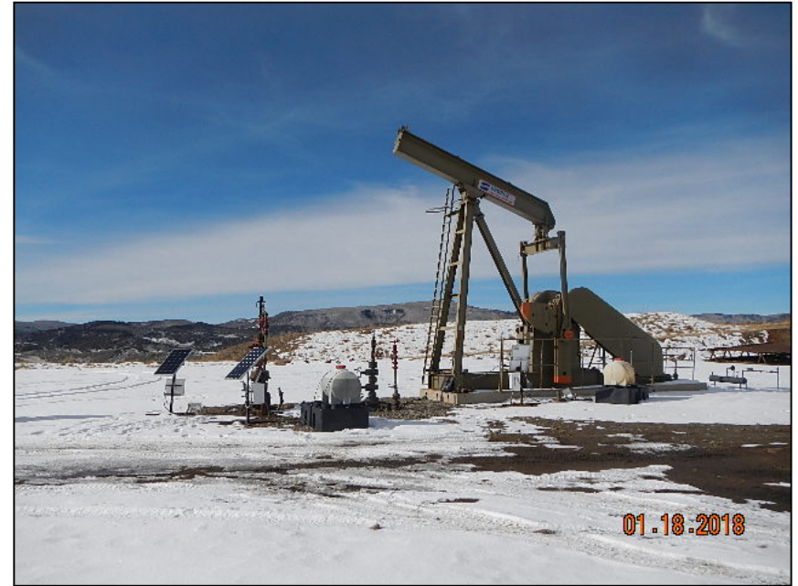
Photo 2. Pump jack disconnected from well.
