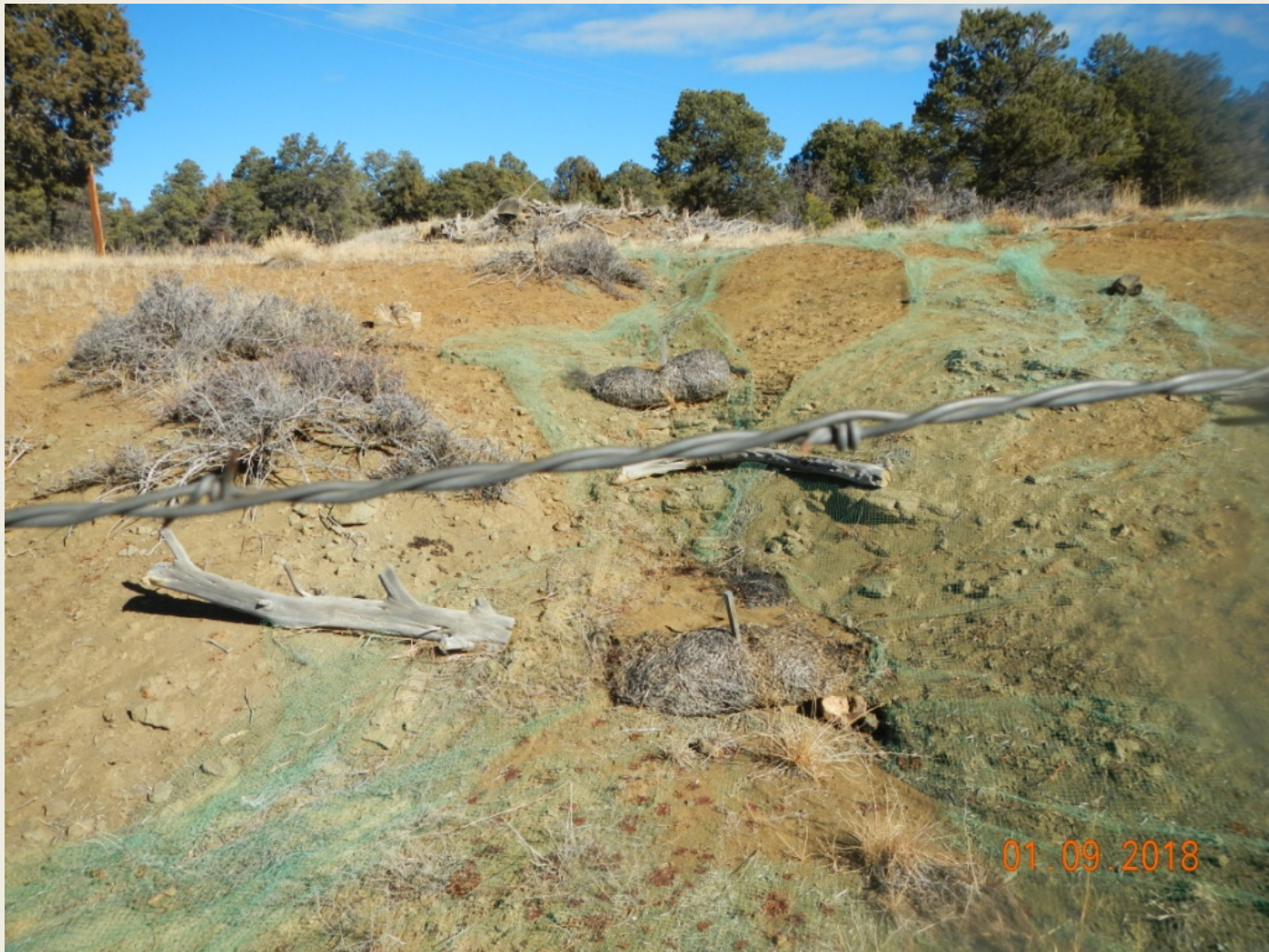
Photo 2. Another view of the northeastern portion of the project area. Wattles are full of sediment and need maintenance. Run-on controls appear needed.
