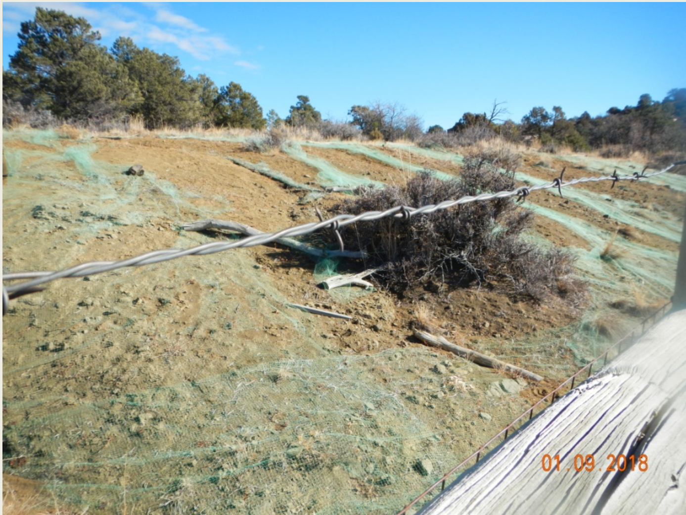
Photo 1. View of the northeastern portion of the project area (cut-slope). Straw blanket for erosion control is no longer functioning. Netting debris needs to be removed and erosion stabilized.
