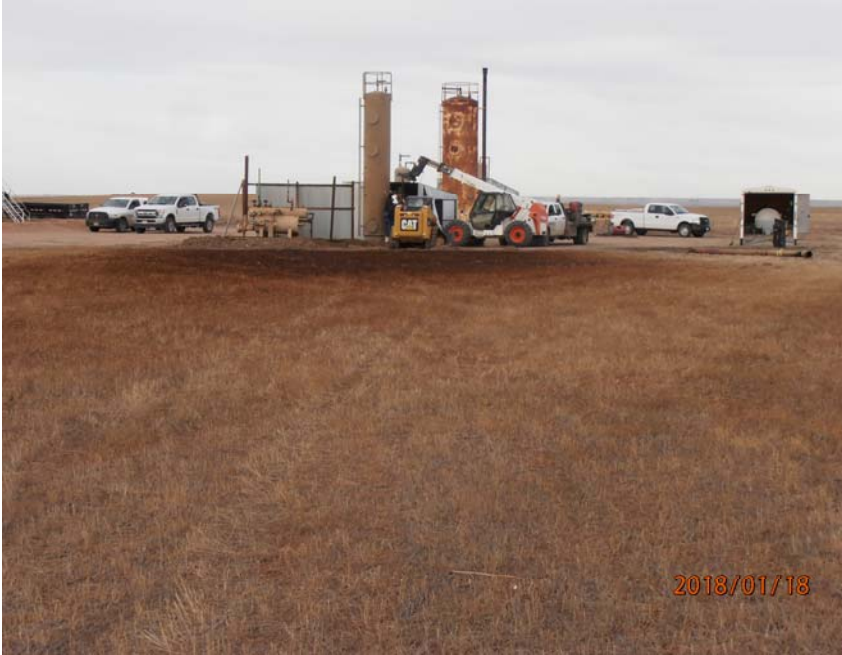
Photo 3 – View of impacted rangeland looking north at heater treater
