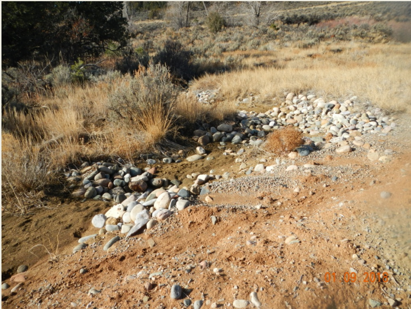
Photo 5. View cobble run-down in the southern portion of the project area. This is filling with sediment and soon require maintenance.
