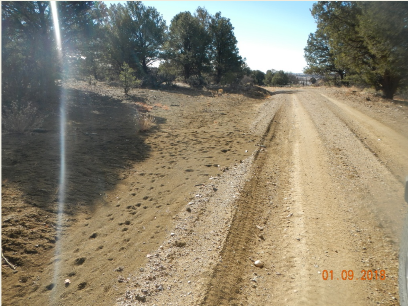
Photo 8. View of roadside drainage full of sediment that needs maintenance.
