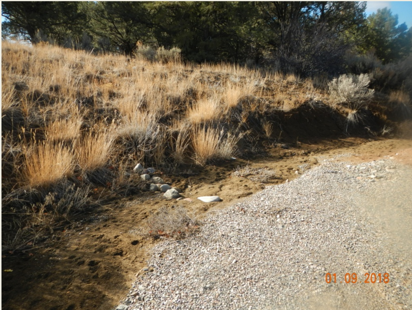
Photo 6. View of cobble check dam and diversion in the southeastern portion of the project area. This is full of sediment and needs maintenance.
