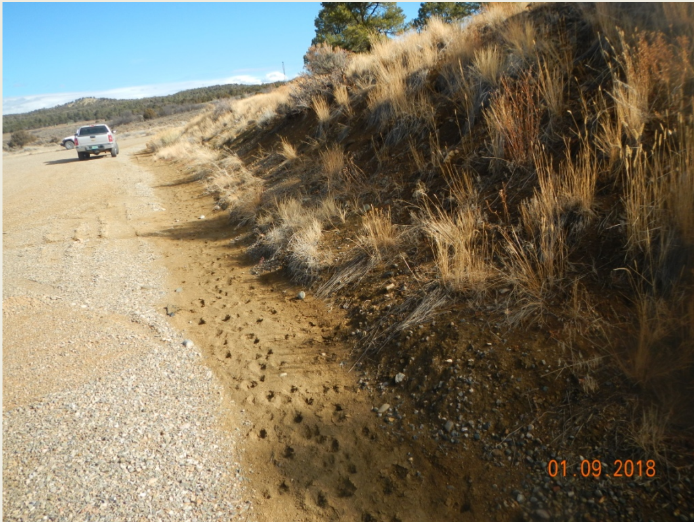
Photo 7. View of diversion in the eastern portion of the project area facing northward. Diversion is full of sediment and needs maintenance.
