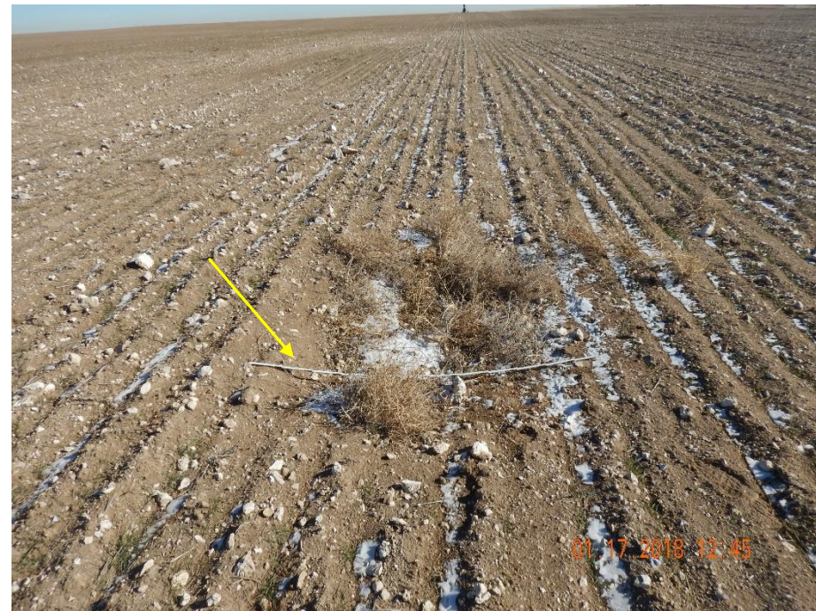
Photo 10: Photo taken from the well on location. Photo shows subsidence concerns remain evident. 6 foot measuring stick (arrow) for reference. Subsidence will need to be repaired.
