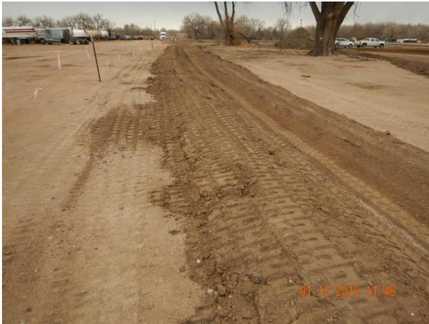
Photo 3. Photo taken from the northwestern location, facing East. Ditch and berm BMP installed.
