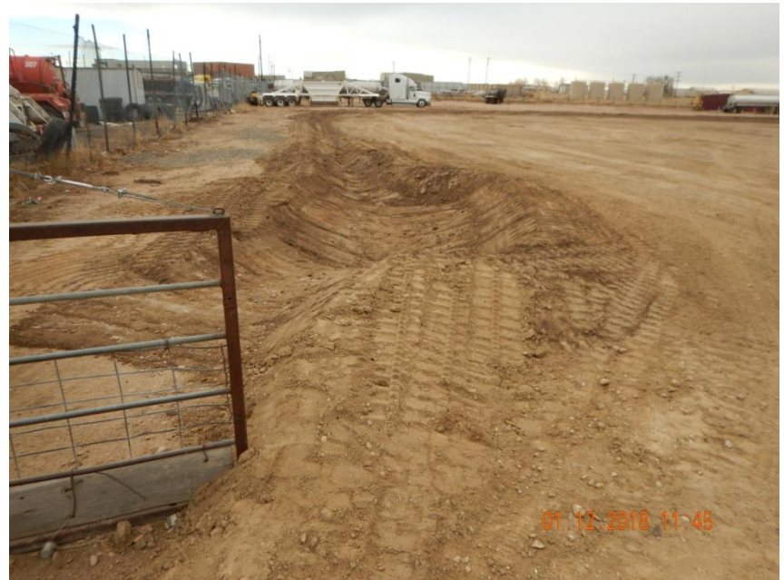
Photo 2. Photo taken from the entrance of location, facing North. Operator IN-PROCESS of constructing what appears to be a sediment trap.
