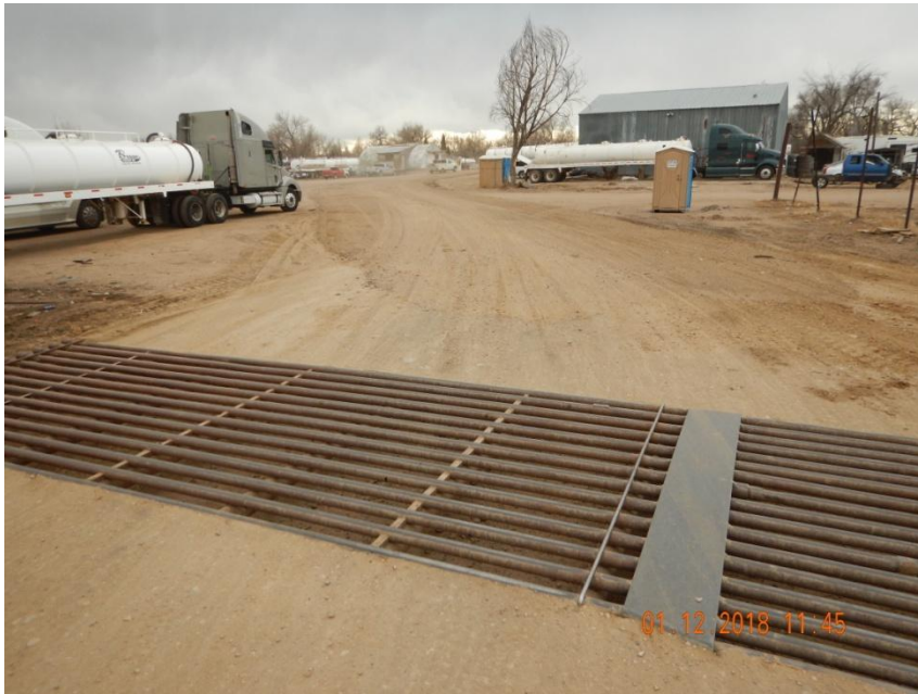
Photo 1. Photo taken from the entrance of location, facing West. Vehicle tracking device installed with road base.
