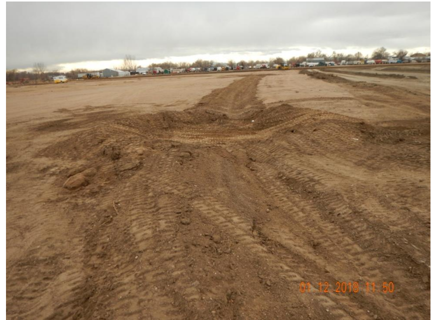
Photo 6. Photo taken from the eastern location, facing West. Operator IN-PROCESS of constructing what appears to be a retention area.
