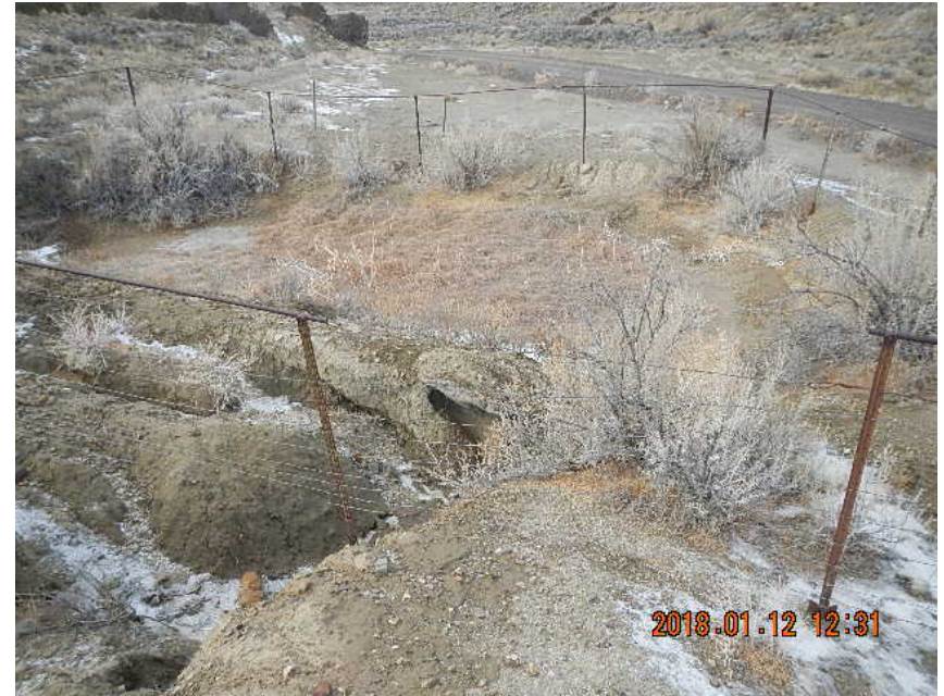
Erosion cuts into blow down pit
