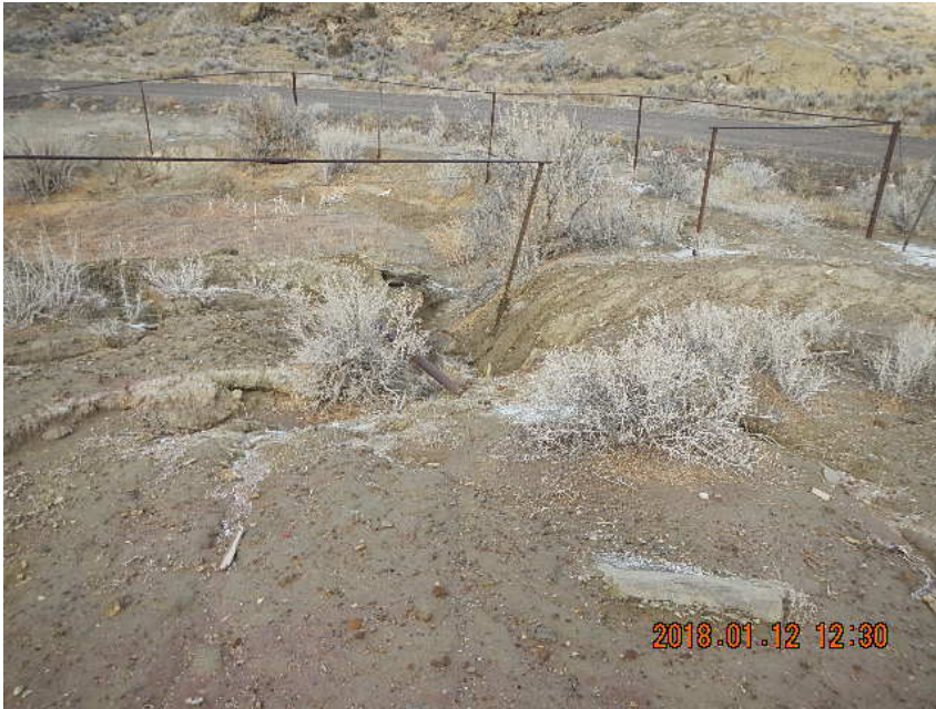
Erosion cuts into blow down pit
