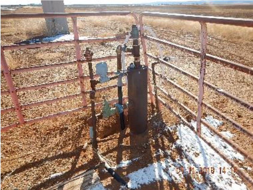
Photo 11: Knockout pot by well pump jack with gas meter shed in background.
