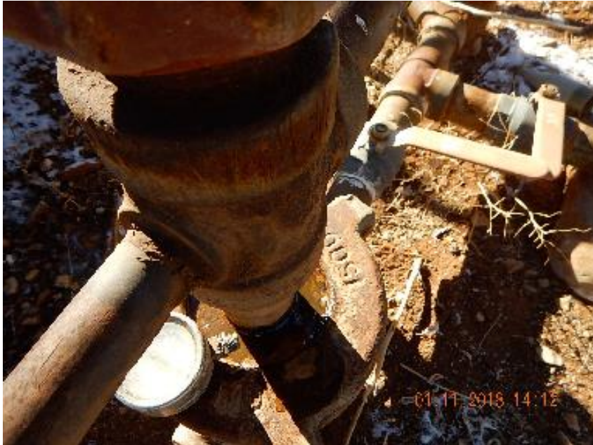
Photo 9: Right side of flange in sunlight are bubbles from venting gas at wellhead flange.
