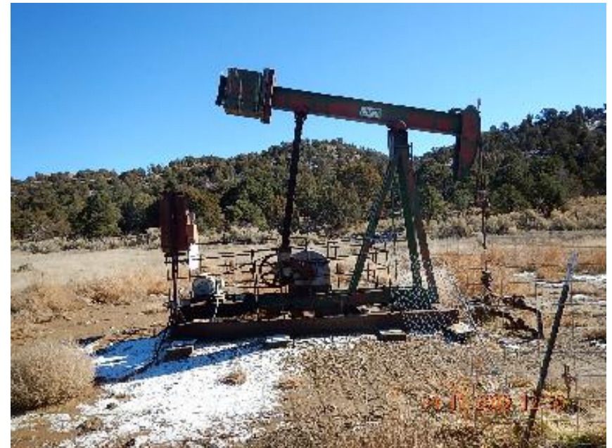
Photo 2: Pump jack, wellhead, and electric panel.
