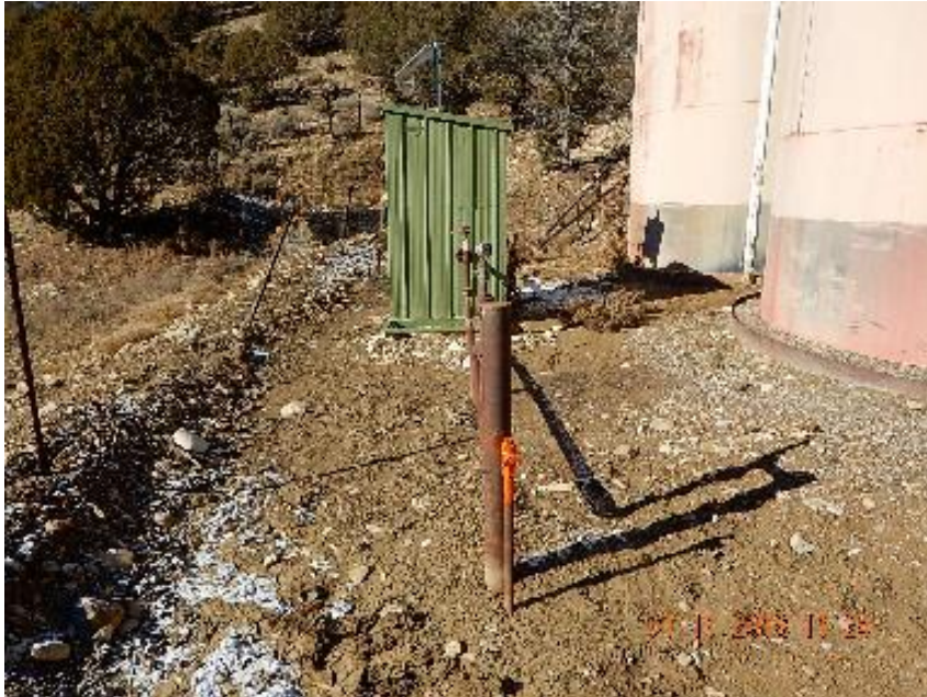
Photo 13: 1" steel riser on W side of tanks out from gas meter run.
