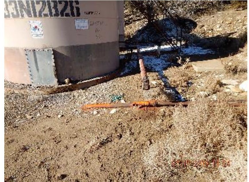
Photo 12: Open ended 3" steel flowline off front of tanks below tank loadout.
