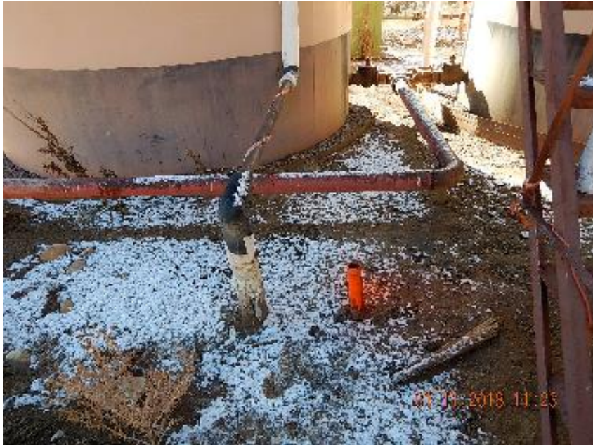
Photo 11: Open ended unused 3" steel riser on E side of tanks.
