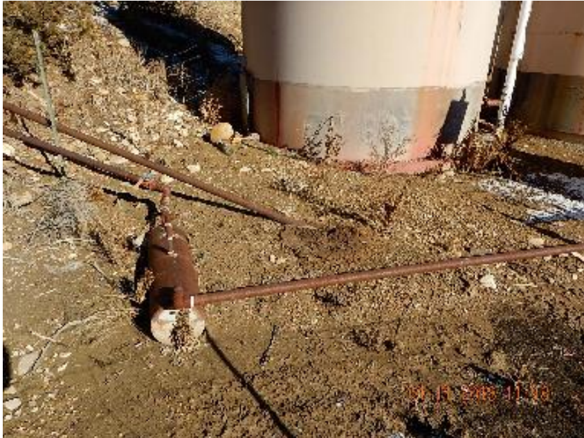
Photo 7: Flowlines at bottom of slope into tank battery. 4" line closest to tank goes into ground but has dried crude oil at surface.
