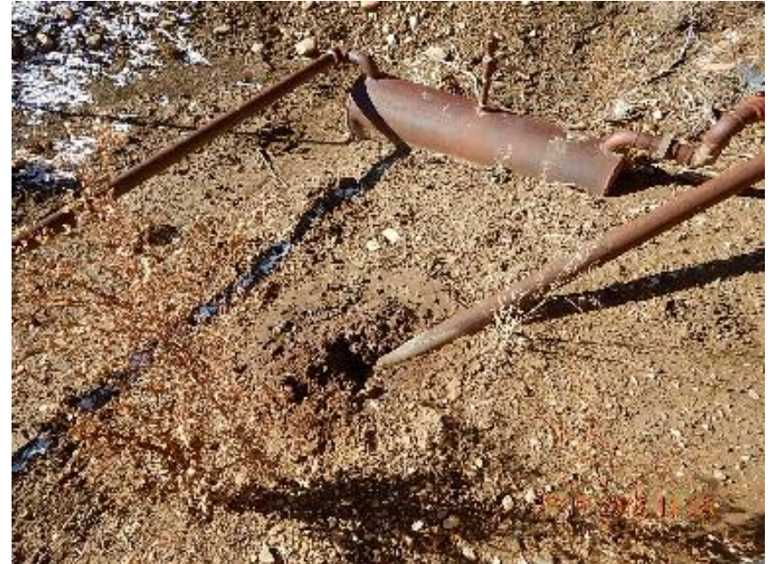
Photo 8: Closer view of 4" line with impacted soil at surface.
