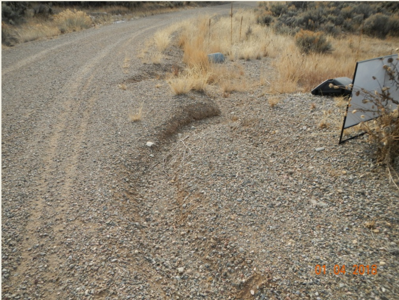
Photo 7. View of erosional channels at the entrance to the well pad.
