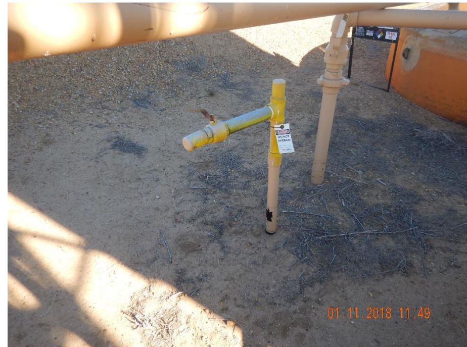
Photo 2: Photo taken from the east end of the battery location. Photo shows pipe riser that has been tagged and painted per the 2017 Flowline NTO, but has not been removed per the NTO required dates. This riser will need to be removed per the NTO and 1004.a.
