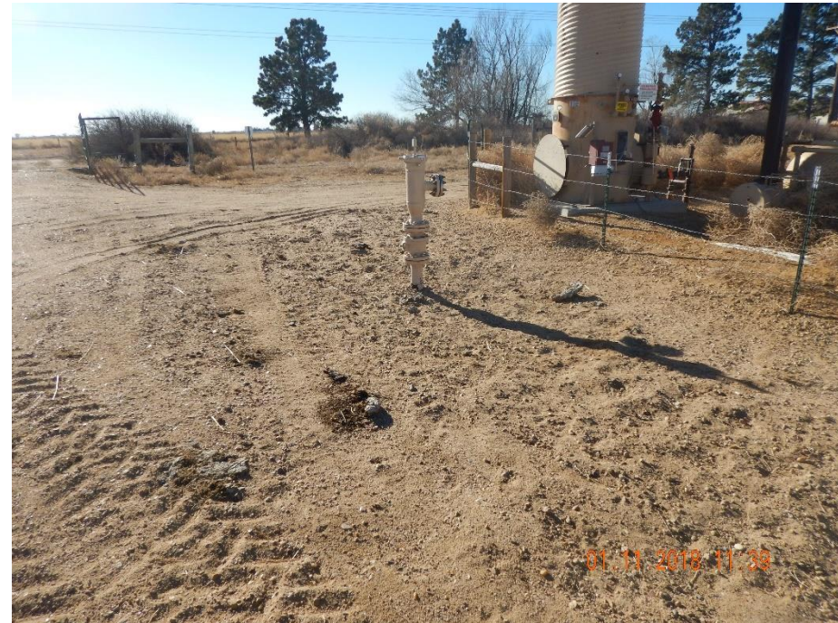
Photo 2: Photo taken from the east end of the battery location, facing south. Previous inspections required operator to removed abandoned riser. Photo shows riser has not been removed.
