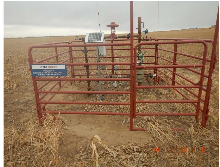
Photo 2: Wellhead, looking N
