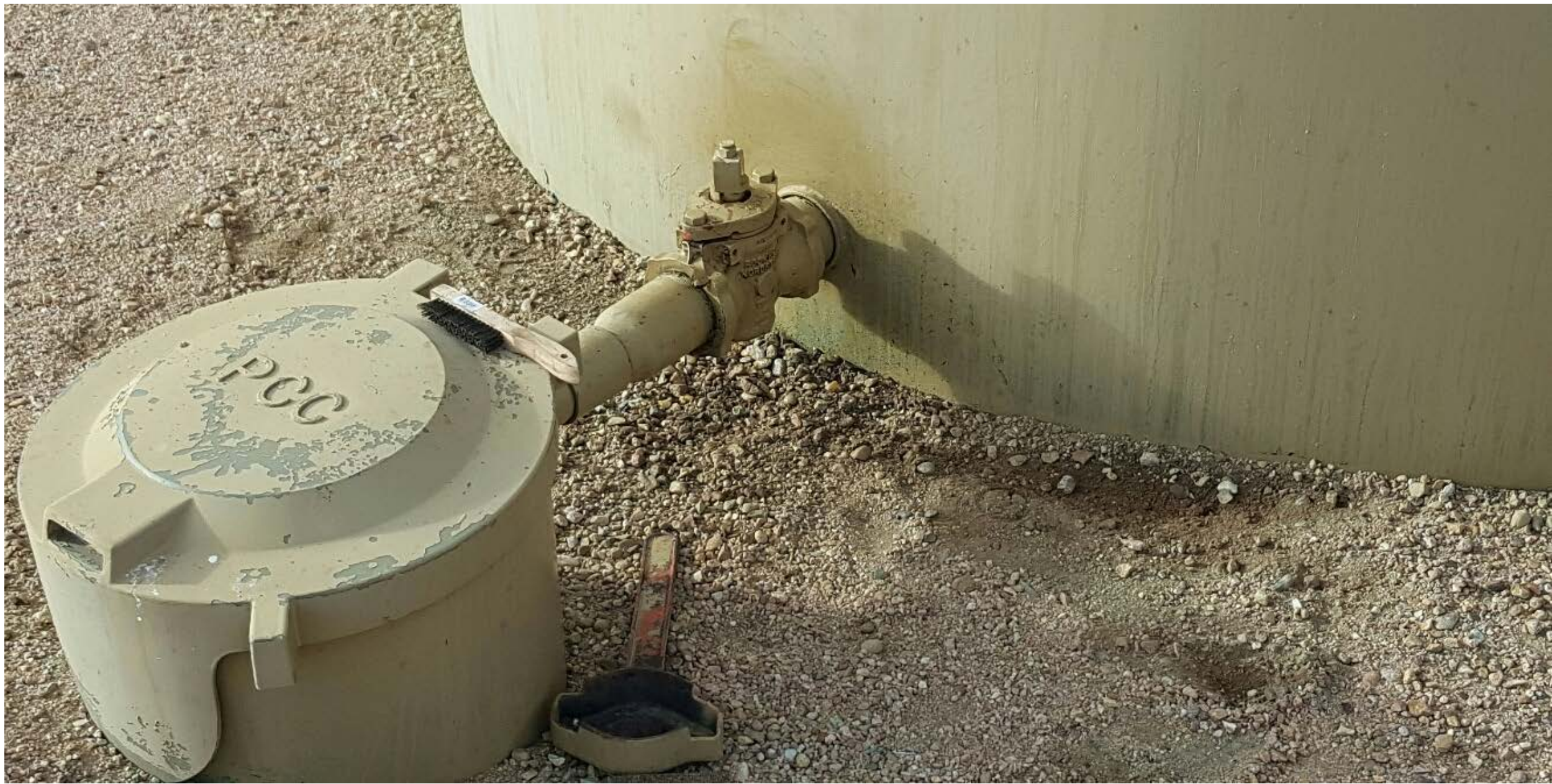
Figure #1 Stained soil under load line removed
