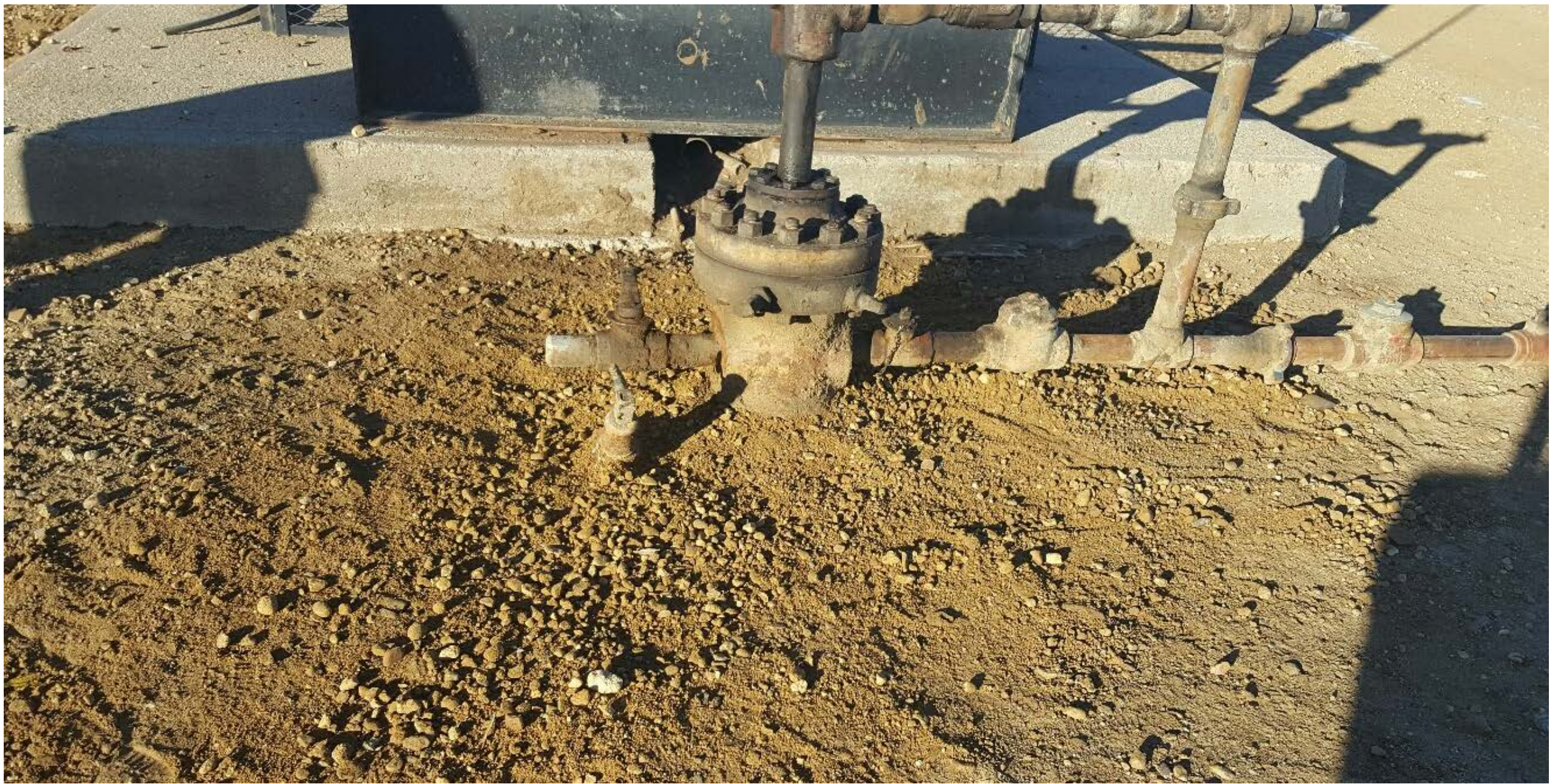
Figure #2 Stained soil and leak have removed
